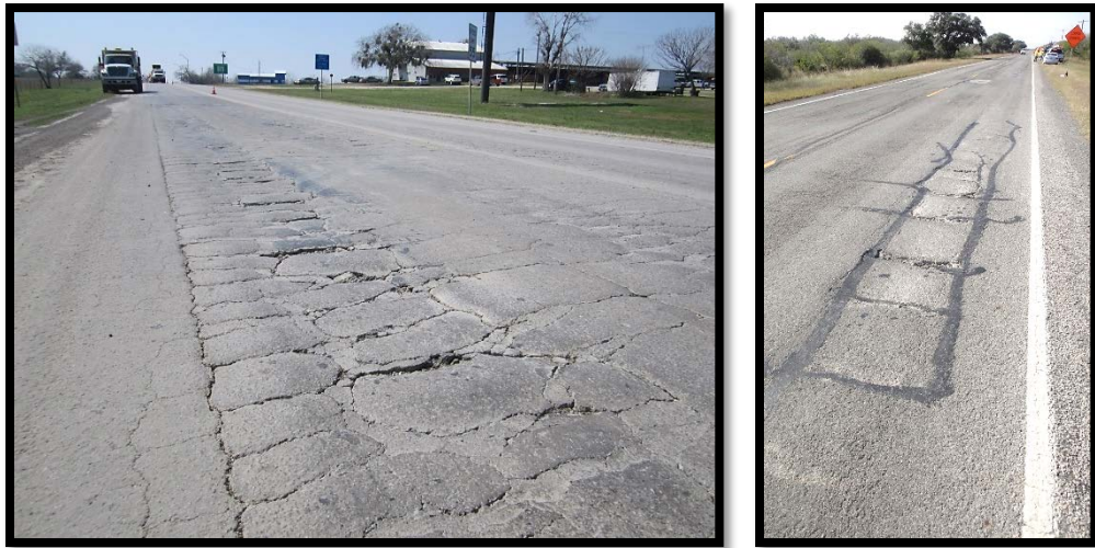
Figure 1. Example Pavements in the Energy Sector Needing Renewal.
