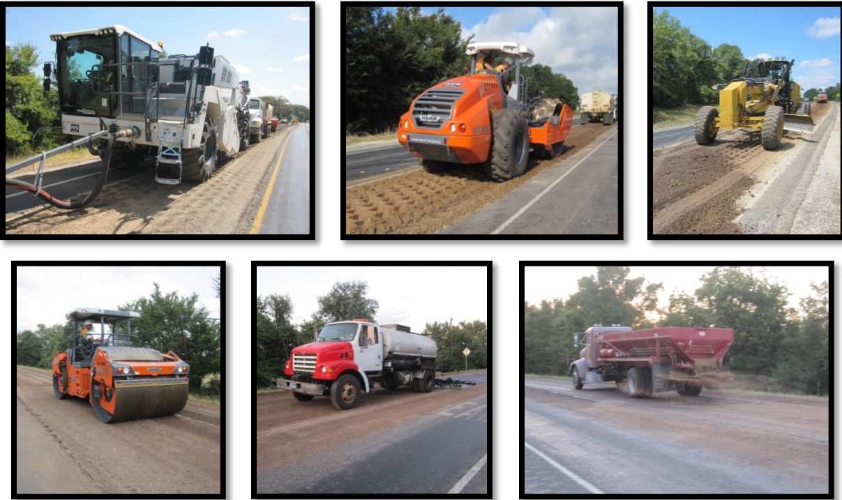
Figure 44. Typical Construction Sequence on SH 7.
