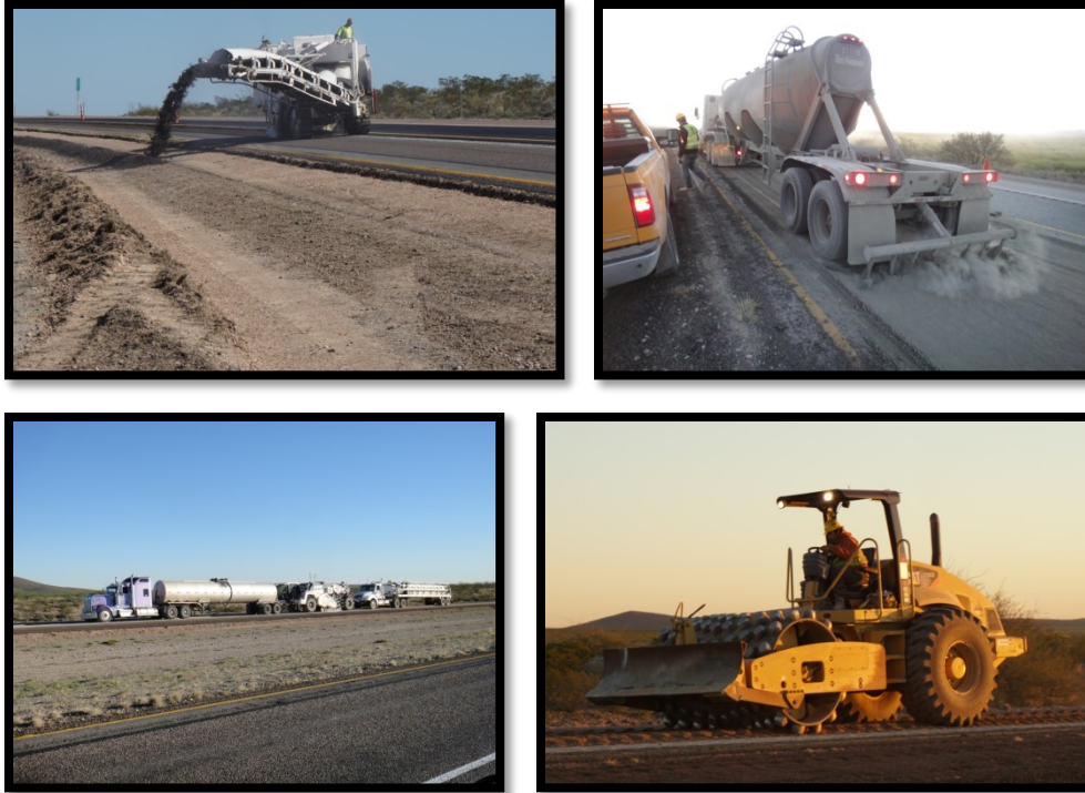
Figure 31. Typical Construction Sequence on IH 10 (Reeves County).
