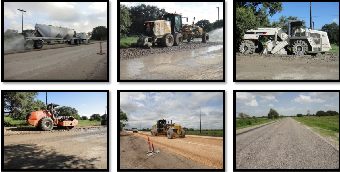
Figure 26. Typical Construction Sequence on SH 202.
