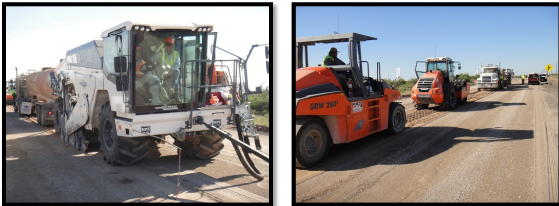
Figure 34. Typical Construction Sequence on SH 115.
