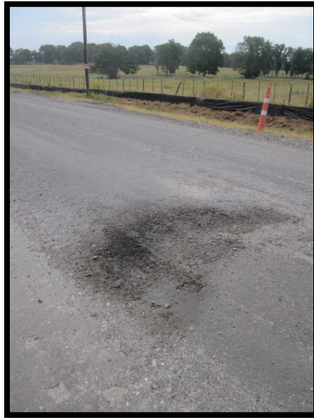
Figure 47. Localized Failure Due to Excessive Water at Location of Disconnecting FDR Train.
