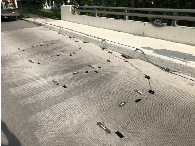
Figure 5. Sensors placed on bridge deck.
