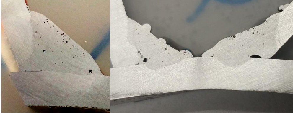
Figure 7: Optical images of weld cross sections from locations in truss distant from observed fractures showing presence of voids within welds
