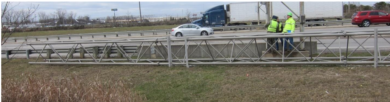
Figure 1: Dismantled truss
