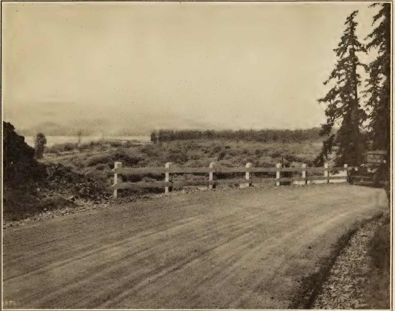
THE GUARD RAIL ERECTED WHERE NEEDED ALONG THE COLUMBIA RIVER HIGHWAY.
