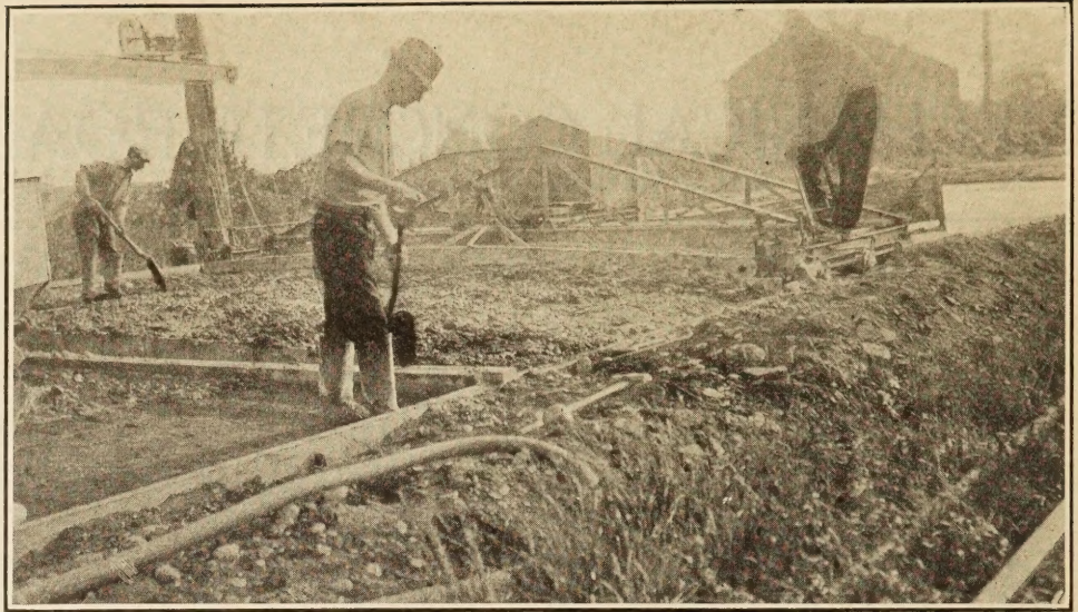
A MIXTURE OF THE PROPER CONSISTENCY. THE MACHINE PERMITS THE USE OF DRIER MIXTURES THAN CAN BE WORKED BY HAND METHODS.
