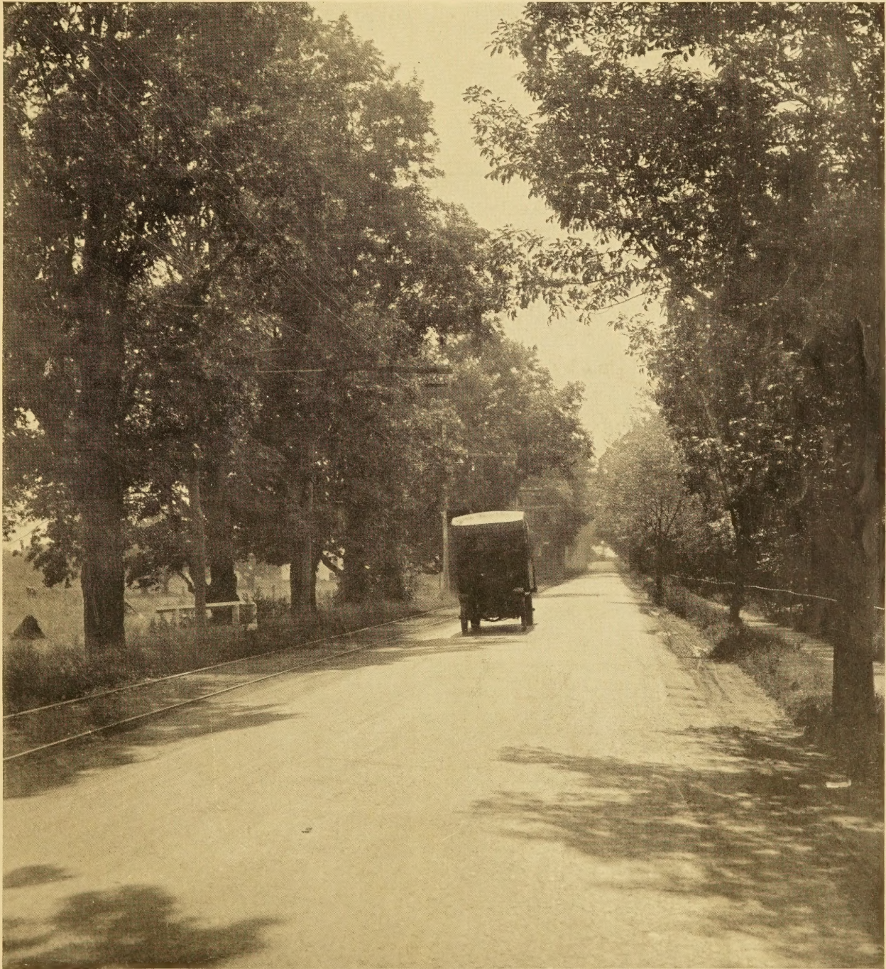
ASPHALT PENETRATION HIGHWAY, MASSACHUSETTS: BUILT 1914
