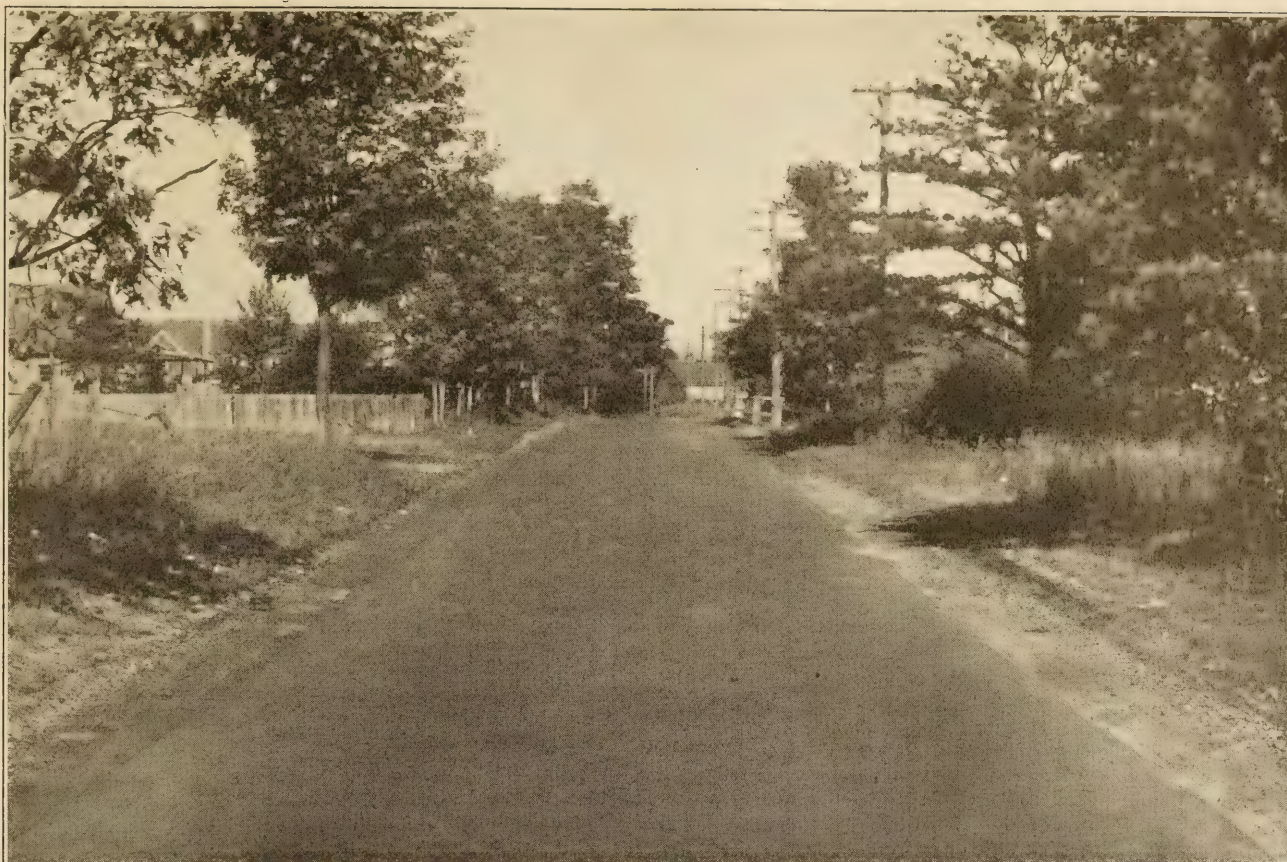
ASPHALT GRAVEL MIX ON GRAVEL BASE NEAR STERLING, MASS., ON MAIN TRUNK LINE TO CAMP DEVENS, MADE IN 1912.
