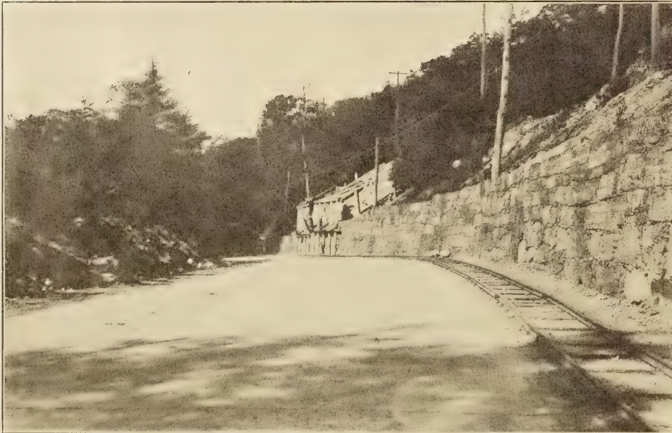
COMPLETED ROAD, NAUGATUCK, CONN., WHICH WAS CONSTRUCTED IN TWO PARTS.
