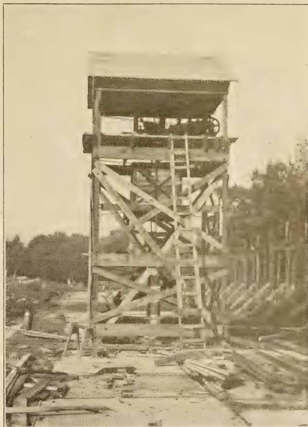
VIEW OF IMPACT MACHINE FOR TESTING ROAD SLABS.
