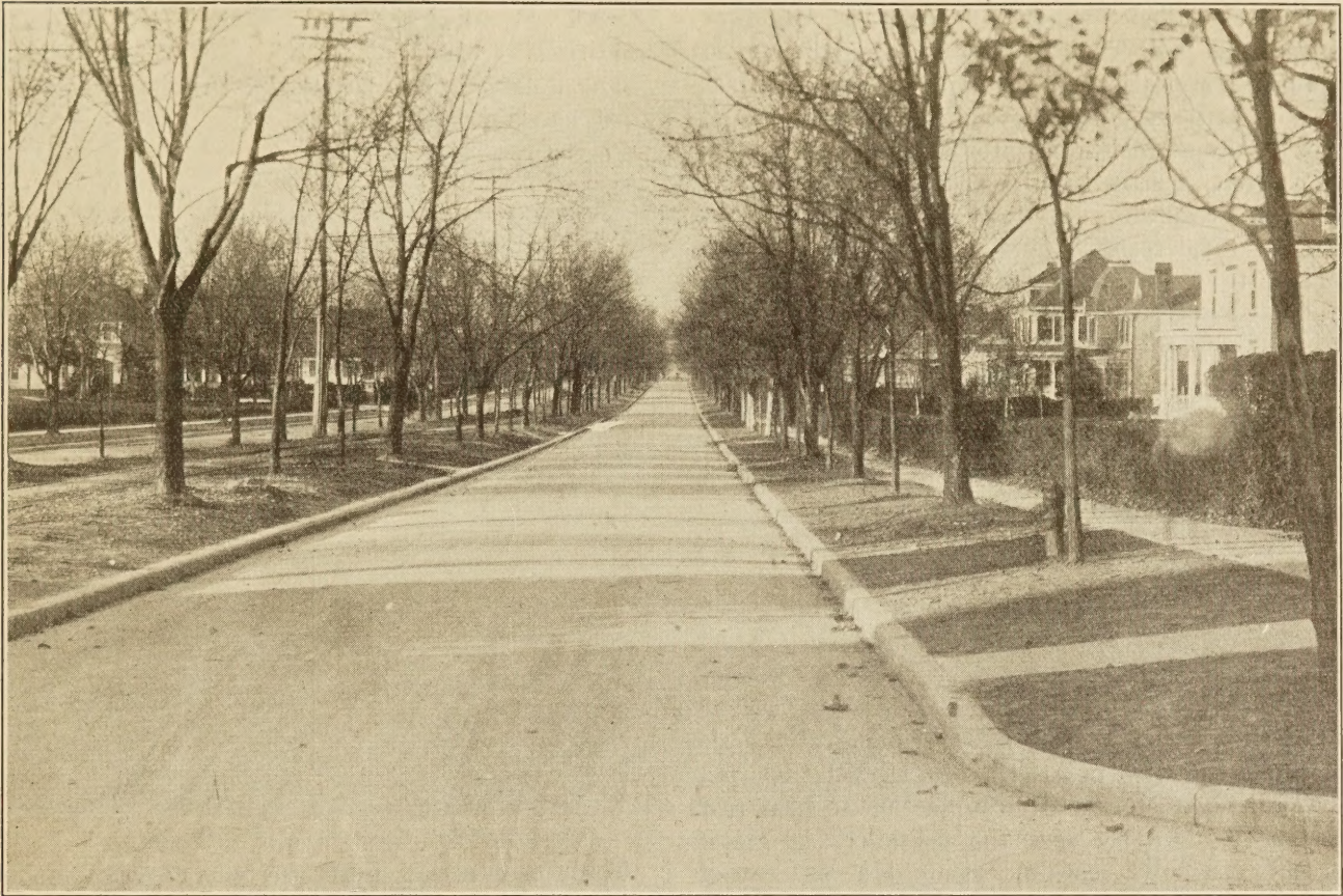
ASPHALT CONCRETE STREET AT NORFOLK, VA., 1914.
