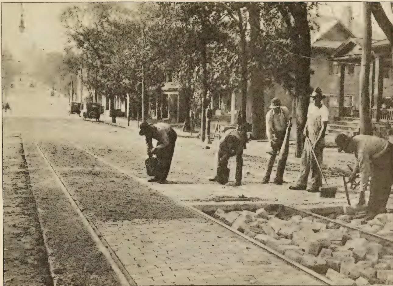
POURING JOINTS WITH ASPHALT FILLER BY POURING-POT METHOD.
