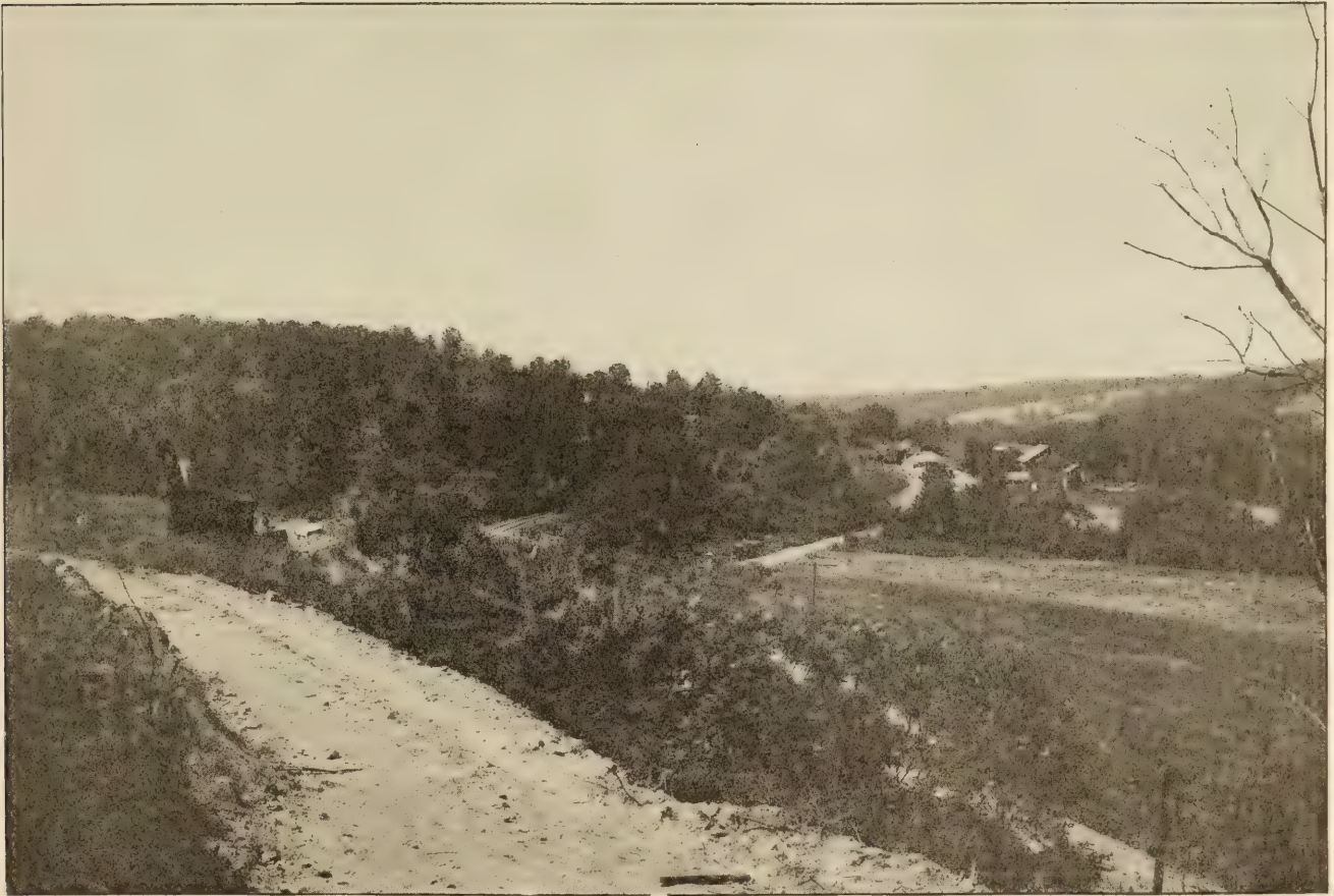
ROAD RELOCATION TO ELIMINATE GRADE CROSSING.
