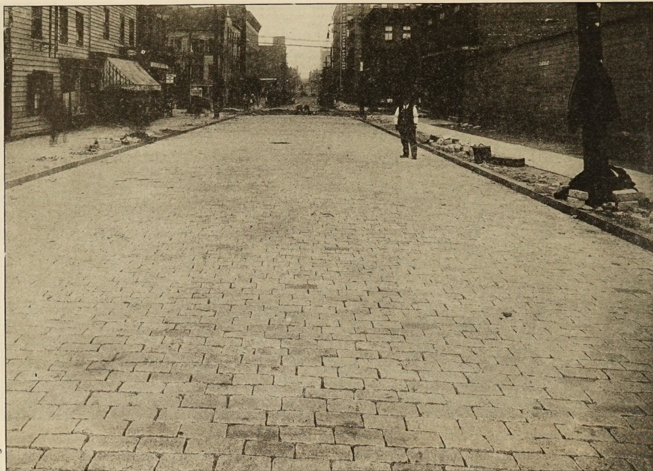
FIVE-INCH GRANITE BLOCKS RAMMED AND READY FOR GROUTING.
