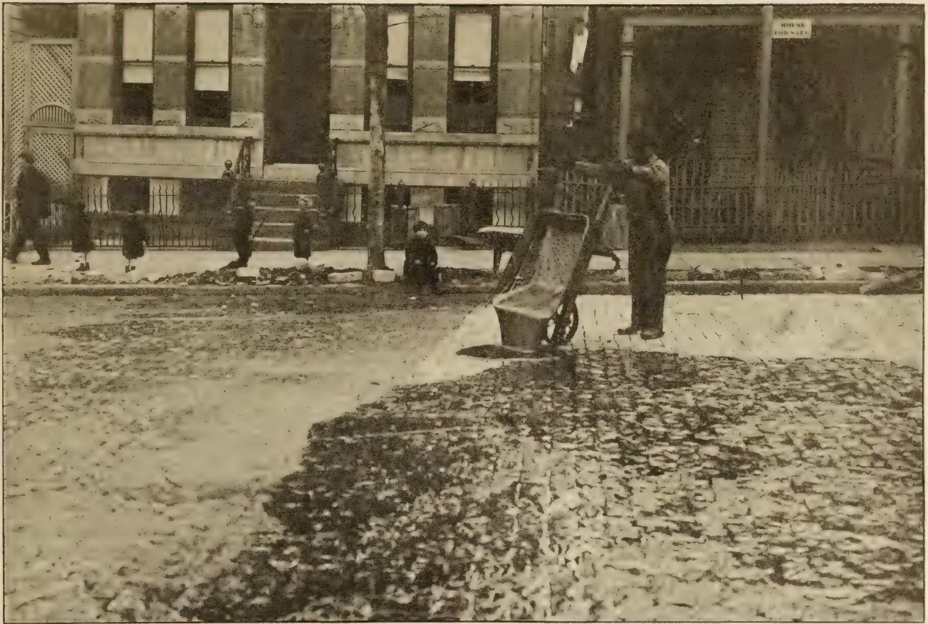
POURING ASPHALT MASTIC FILLER COMPOSED OF ONE PART ASPHALT AND ONE PART SAND.
