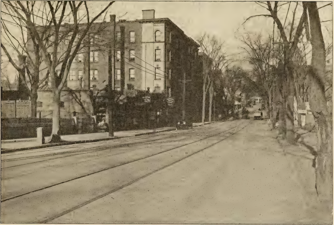
GRANITE BLOCK, GROUTED WITH 1 TO 1 CEMENT GROUT, WORN SMOOTH BY TRAFFIC.
