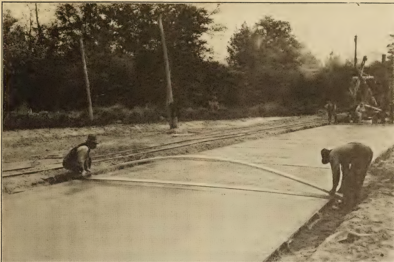
USING THE SPECIALLY DEvised 10-INCH BOW BELT ON DELAWARE FEDERAL AID PROJECT NO. 4.
