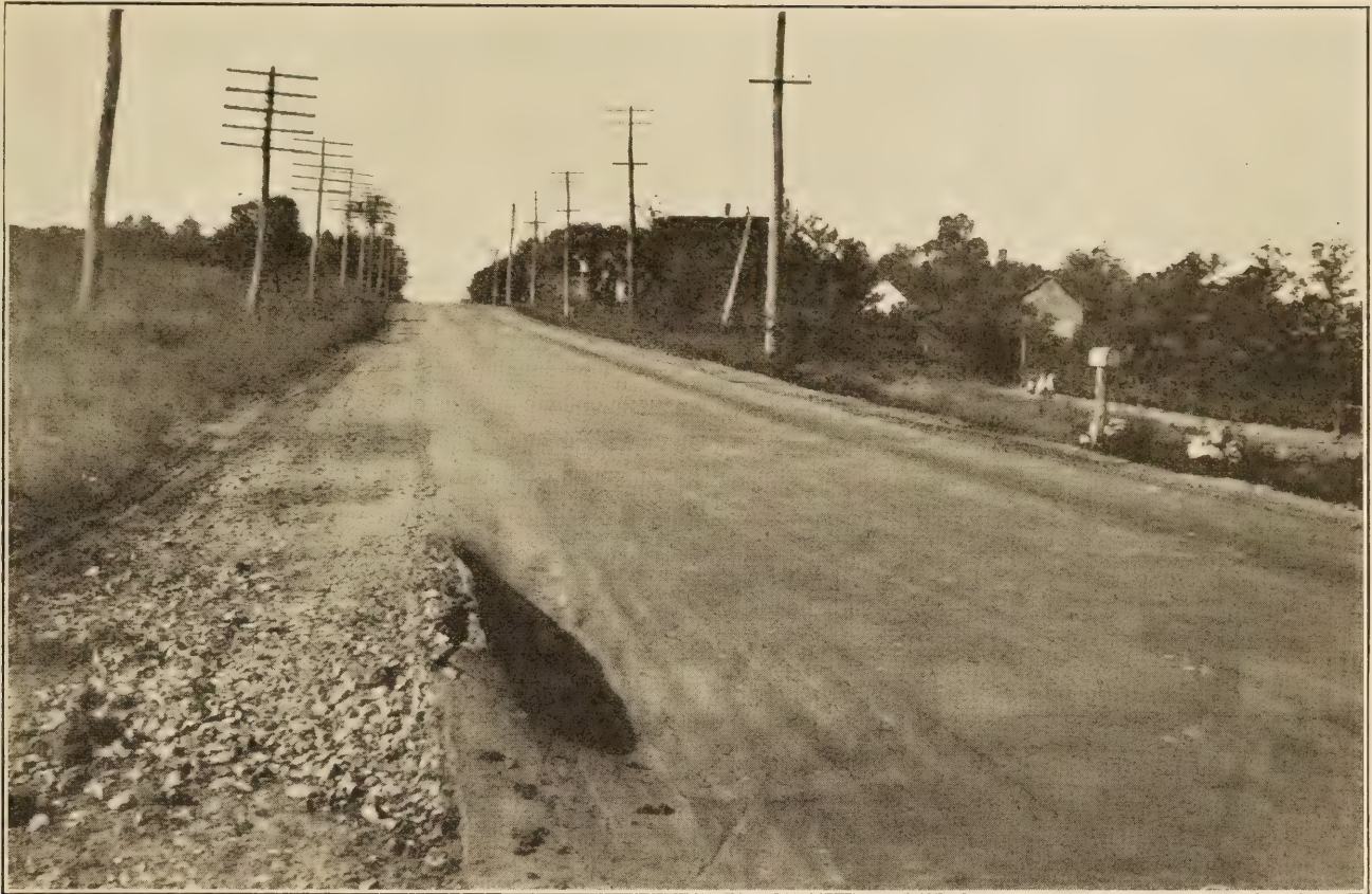
FAILURE DUE TO A SATURATED CLAY SPOT UNDER A BITUMINOUS CONCRETE ROAD IN NEW JERSEY. THIS HOLE IS SO DEEP THAT THE TRUCK AXLES HAVE RAKED THE BUNCH AT THE LEFT OFF FLAT.
