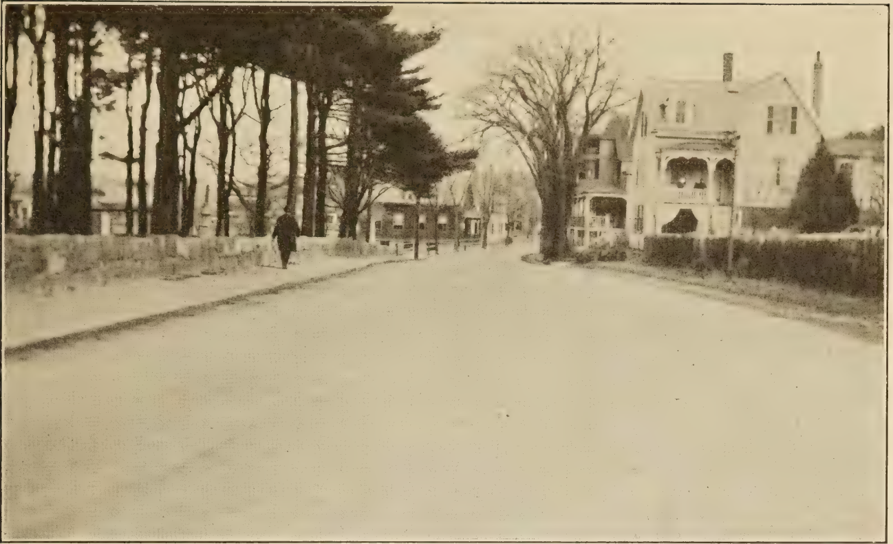
MANCHESTER, MASS., ASPHALT PENETRATION ROAD LAID IN 1916. PHOTOGRAPH WAS TAKEN IN MARCH, 1919.
