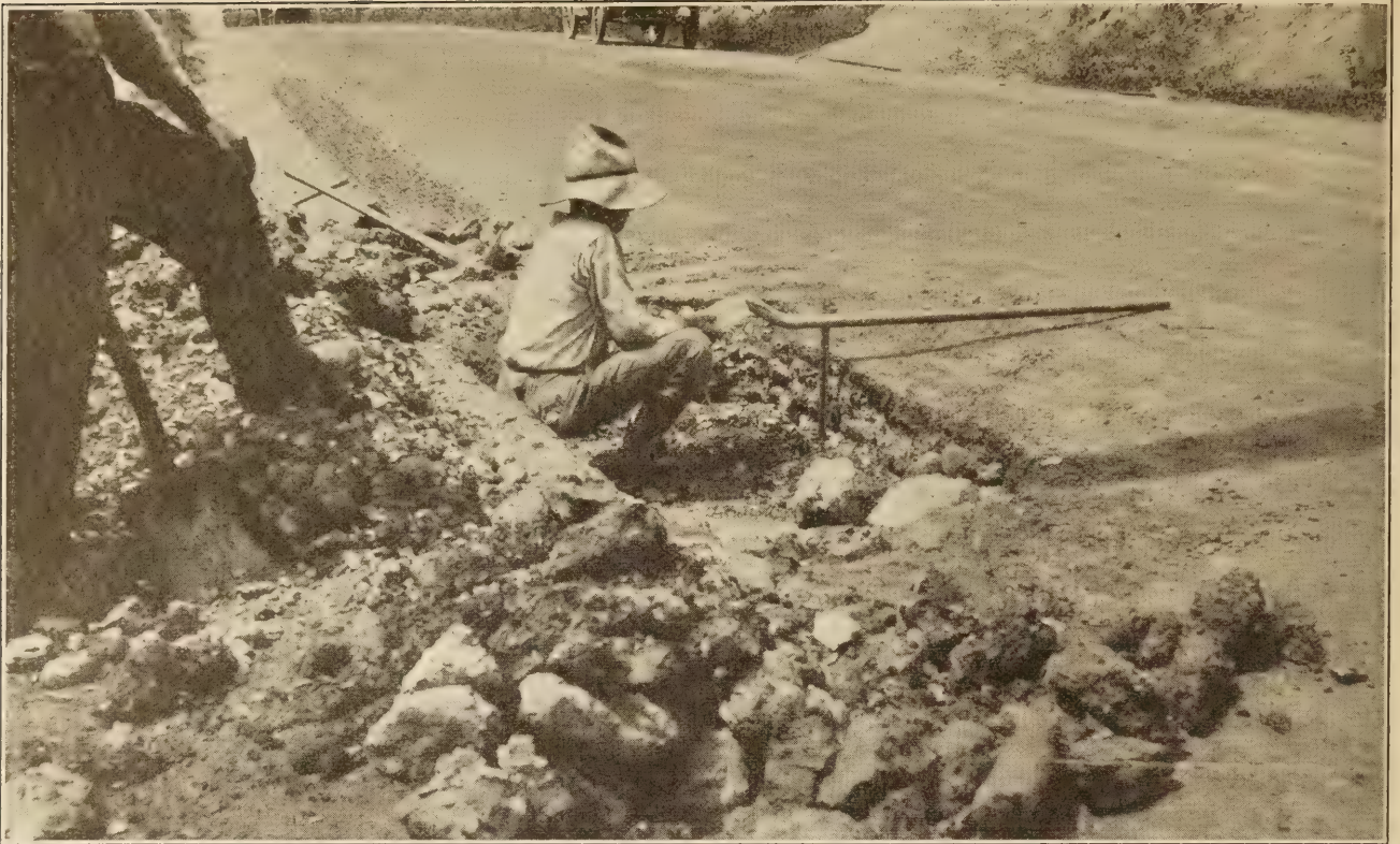
BITUMINOUS CONCRETE ON A PORTLAND CEMENT CONCRETE BASE. WET CLAY WAS FOUND UNDER THIS BREAK. END OF SHOVEL HELD BY THE BOY SHOWS WHERE THE PAVEMENT SURFACE LAY ORIGINALLY AND DEMONSTRATES THE FACT THAT WET CLAY IS A POOR FOUNDATION. THIS SPOT IS ON A HILL, WELL DRAINED, BUT SEEPAGE THROUGH THE SHOULDERS KEPT THE CLAY MASS WET.
