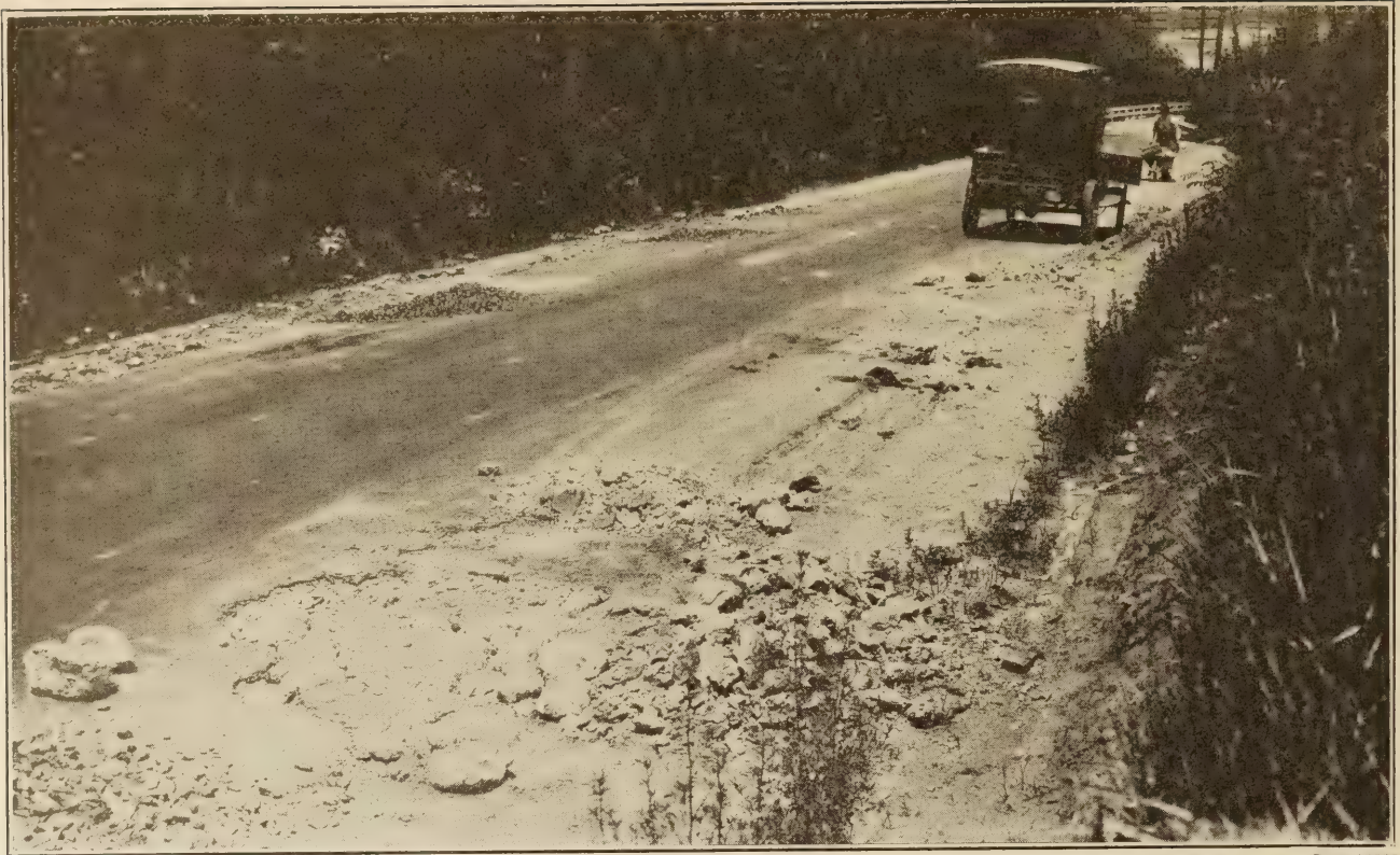
THE BREAKS IN PROCESS OF REPAIR OCCURRED OVER POCKETS OF CLAY WHICH ABSORBED AND RETAINED ENOUGH WATER TO KEEP THE CLAY PLASTIC.
