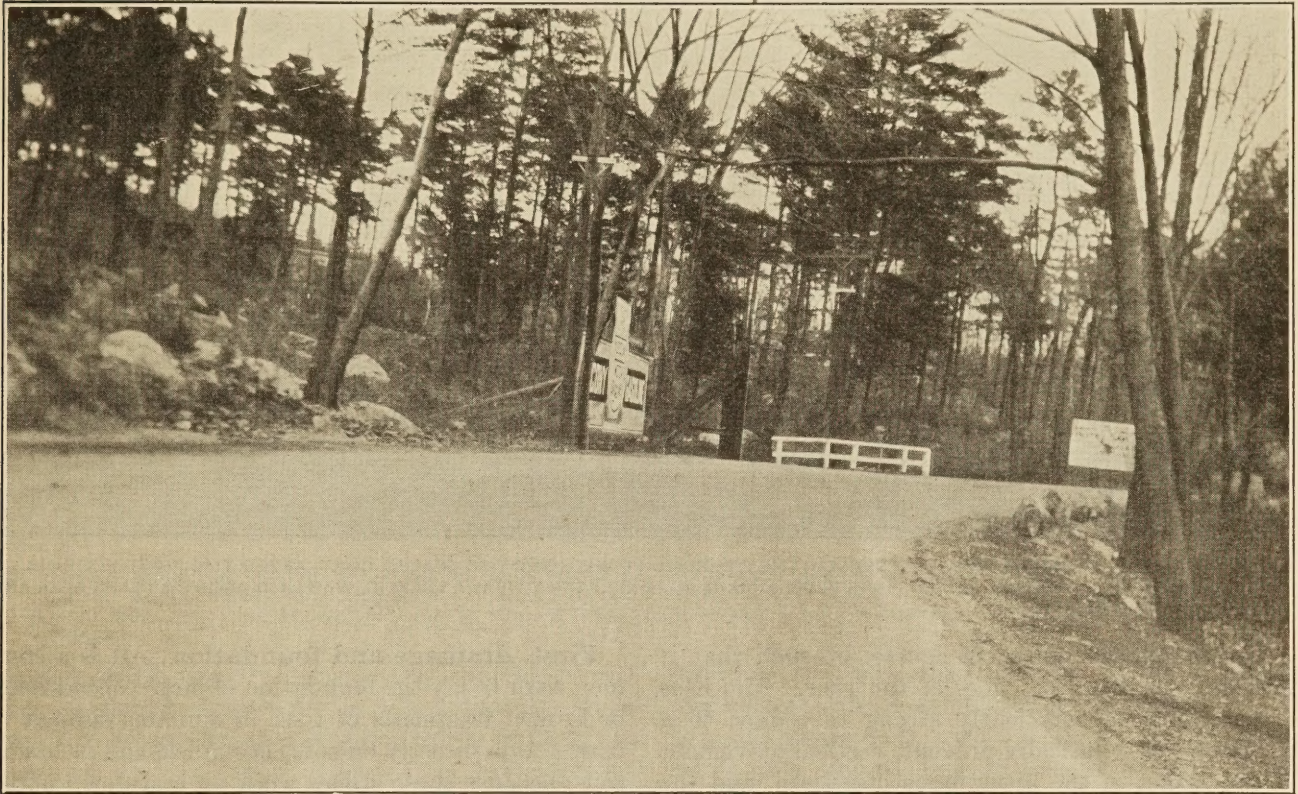
GLOUCESTER, MASS., SHOWING BANKED CURVE ON STATE ROAD RECONSTRUCTED IN 1917. THE BINDER WAS ASPHALT. THE PHOTOGRAPH WAS TAKEN IN MARCH, 1919.
