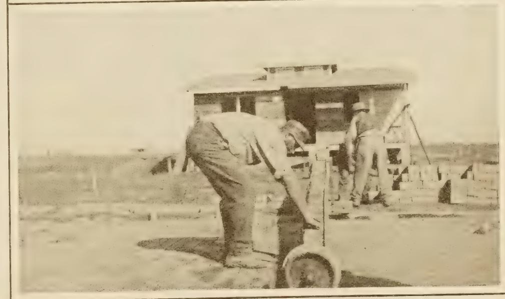
CONSTRUCTION OF A FEDERAL AID BRICK ROAD IN NEBRASKA. TOP—LAYING CONCRETE BASE. CENTER—SPREADING SAND CUSHION. BOTTOM—LAYING THE BRICK.
