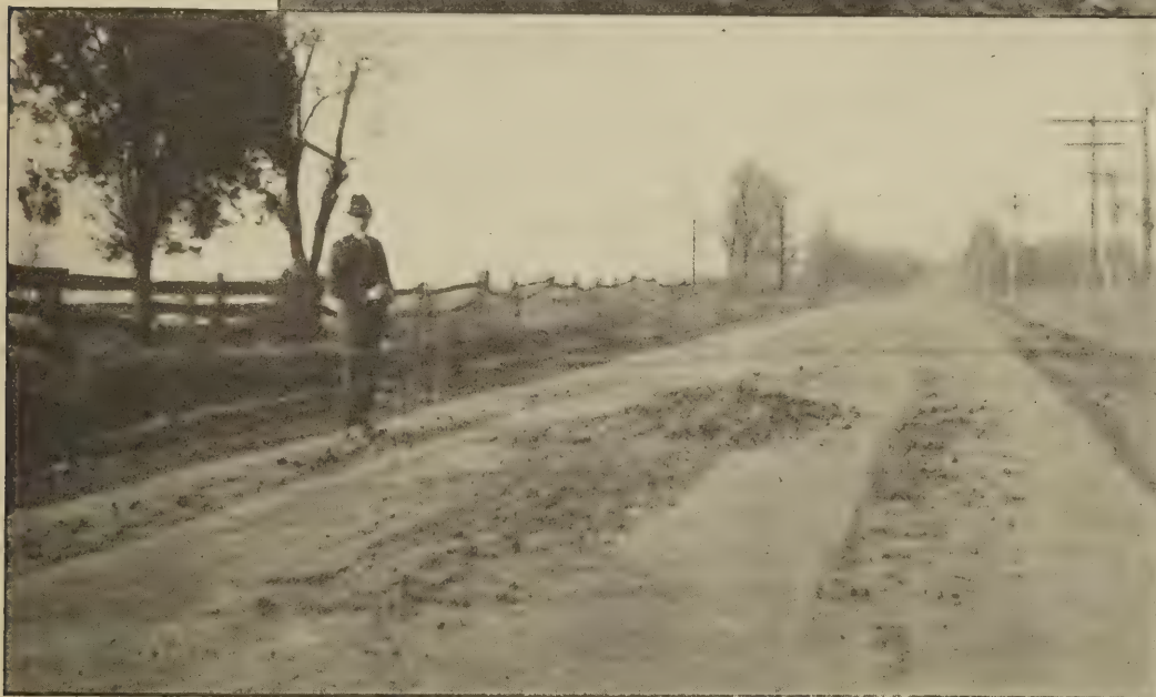
BITUMINOUS CONCRETE ROAD ON THE PHILADELPHIA-NEW YORK MAIN LINE BETWEEN NEW BRUNSWICK AND HIGHTSTOWN N. J. THIS ROAD WAS BUILT IN 1918.
