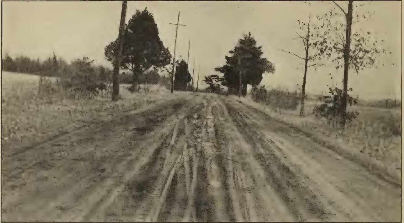
WATER-BOUND MACADAM, OIL SURFACE TREATMENT, AT WAYLAND, MASS. SURFACING 8 INCHES, BLANKET COAT 90 PER CENT HOT OIL ONE-HALF GALLON PER SQUARE YARD IN 1910, ONE-HALF GALLON HOT TAR PER SQUARE YARD 1909. REBUILT IN 1916, BERMUDEZ ASPHALT PENETRATION, 5 INCHES BROKEN STONE BASE OVER 12 INCH GRAVEL FOUNDATION, WITH 2 1-2 INCH BERMUDEZ ASPHALT TOP.
