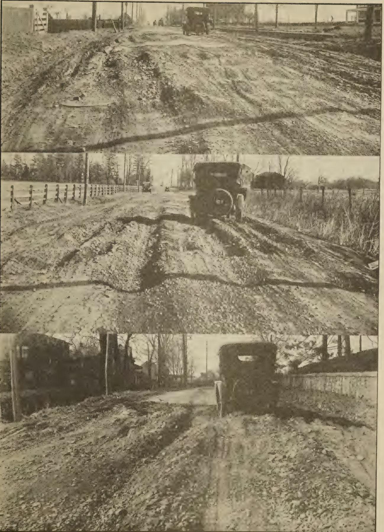
ON THE PHILADELPHIA PIKE. FROM TOP TO BOTTOM, 1, 2, AND 4 MILES NORTH OF WILMINGTON, DEL., MACADAM SURFACED, 18 FEET, WITH BITUMINOUS MATERIAL, 1914. SUBGRADE—SAND—ROCK—CLAY. DRAINAGE GOOD. THIS ROAD CARRIED THE ORDINARY TRAFFIC WITH MODERATE MAINTENANCE. ITS CONDITION AS SHOWN IS THE RESULT OF THE PASSAGE OF A FLEET OF 100 HEAVY TRUCKS.
