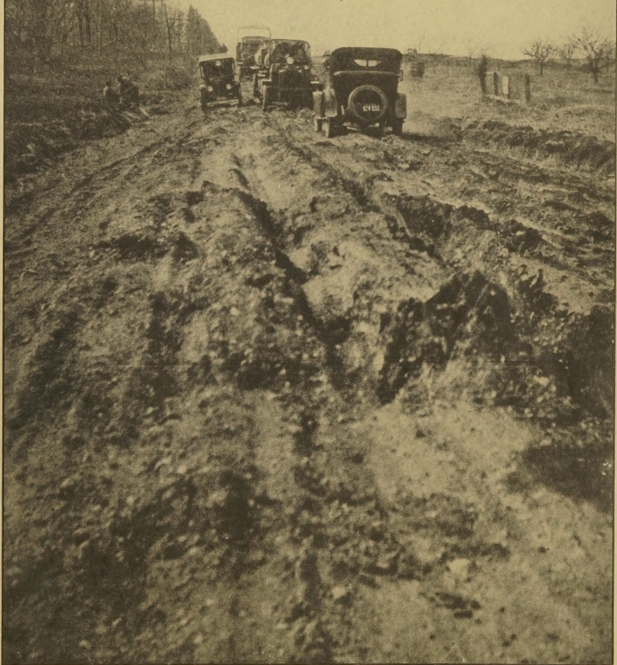
THIS PHOTOGRAPH WAS TAKEN NEAR CANANDAIGUA, N. Y., AND SHOWS WHAT AN EXCESS OF ABOUT THIRTY 7-TON UNITS ABOVE NORMAL TRAFFIC CAN DO TO A MODERN HARD-SURFACED HIGHWAY. ABOUT ONE AND A HALF MILES OF THIS ROAD IS IN LIKE CONDITION
