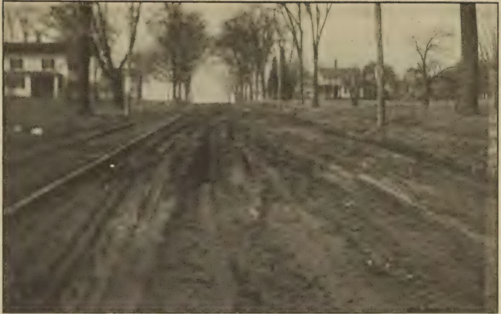
ON THE BERLIN TURNPIKE, BETWEEN HARTFORD AND MERIDEN, CONN. THIS ROAD HAS BEEN CALLED UPON TO CARRY 200 5-TON TRUCKS PER DAY. THE RESULT IS SHOWN.
