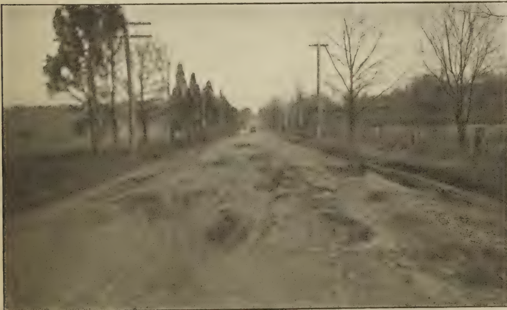
THIS HIGHWAY, BETWEEN WATERBURY AND SOUTHINGTON, CONN., BEARS A DAILY TRAFFIC OF 2,500 VEHICLES, OF WHICH ABOUT 250 ARE HEAVY UNITS.
