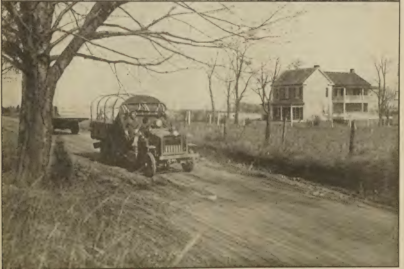
ONE OF THE EXPERIMENTAL ROADS IN THE VICINITY OF WASHINGTON—THE ALEXANDRIA-GUM SPRING ROAD—SHOWING EARLY FAILURES AND CHARACTER OF TRAFFIC THAT CAUSED THEM.
