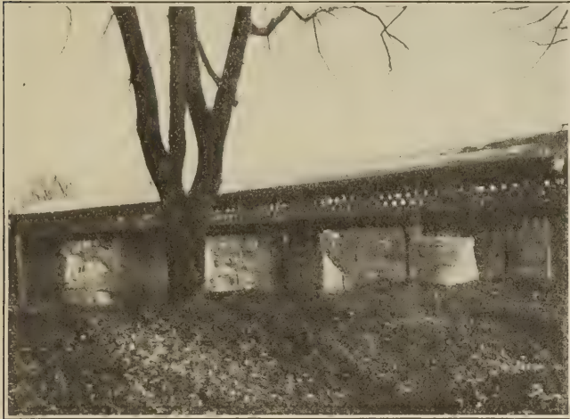
Old covered wooden bridge replaced with modern steel truss type of construction by Michigan State Highway Department.
