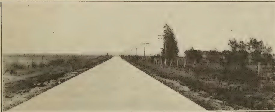
Completed concrete paving in Iowa. Shoulders not finished.
