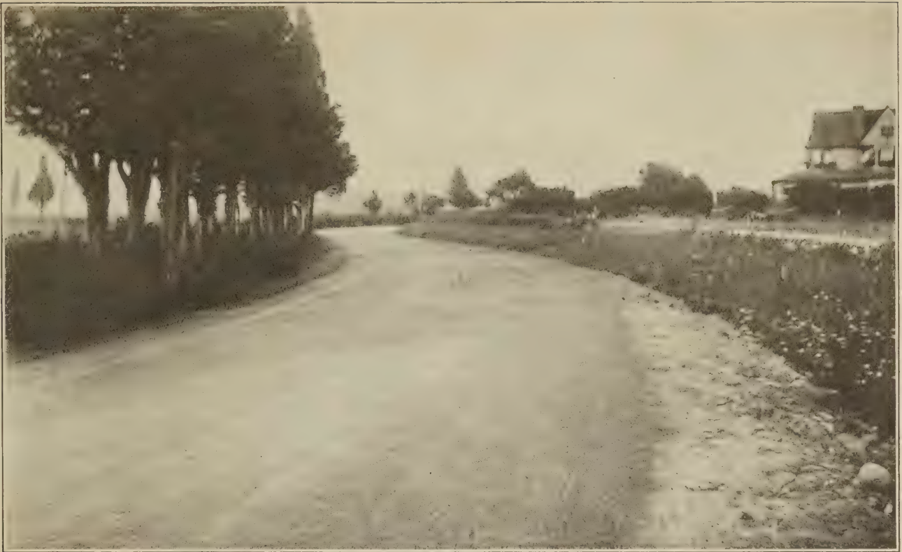
Reverse curve on a Rhode Island highway, showing one-way slopes on curves.
