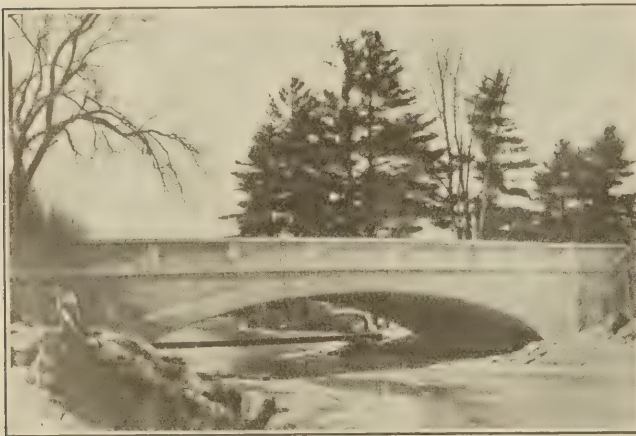
Concrete arch bridge, Rhode Island.
