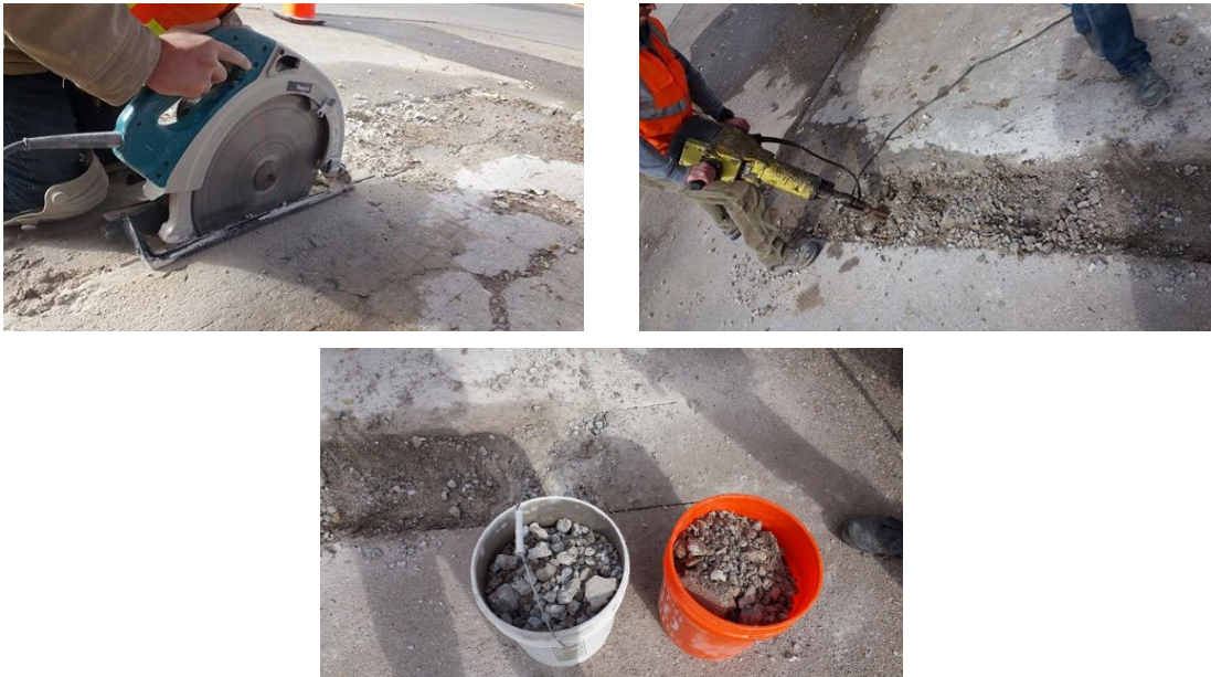
Figure 3.1 Process of collecting RCA aggregates
