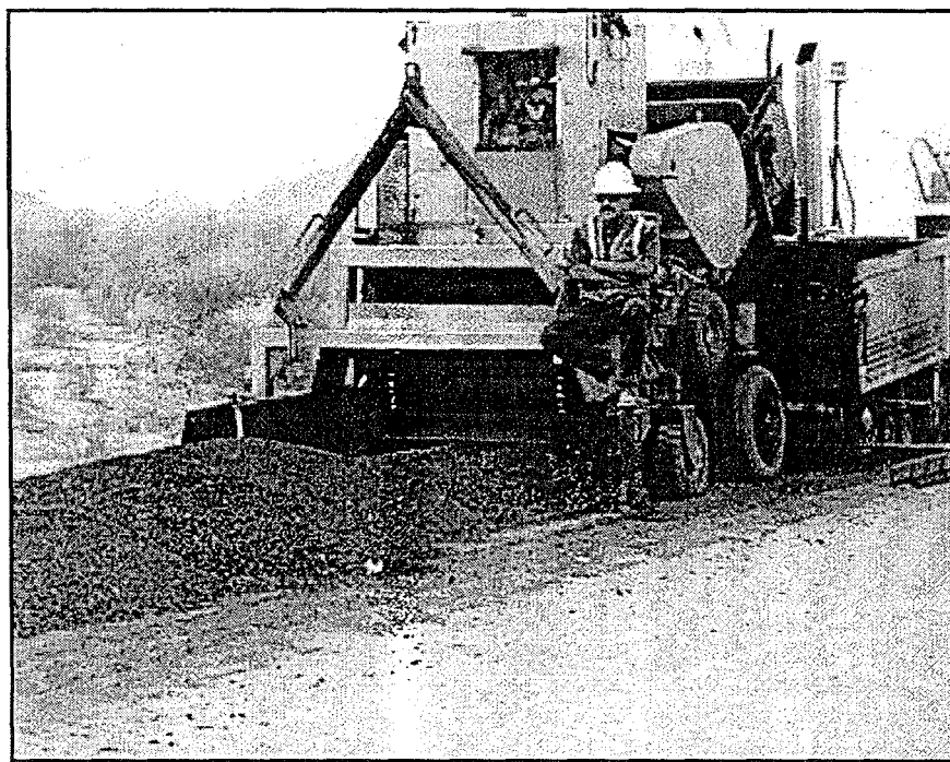
Figure I.6. Cold In-Place Recycled Windrow Behind Paver
