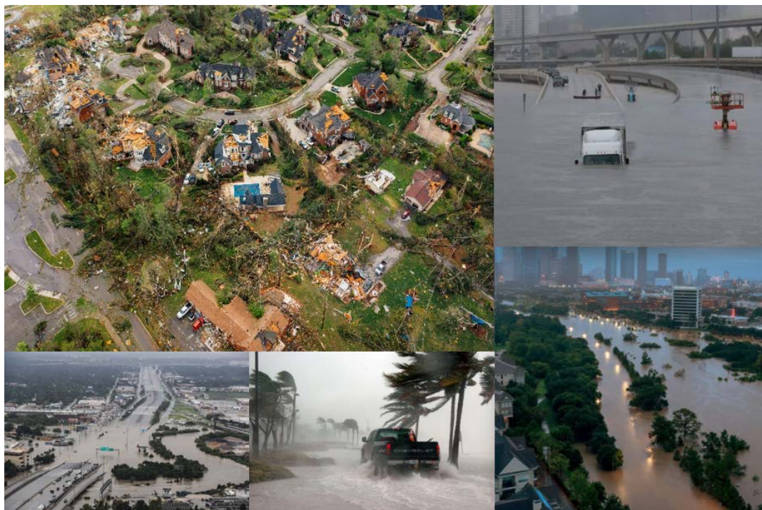
Figure 2. Hurricane Harvey damages in Houston in 2017 (web sources 1 2).
