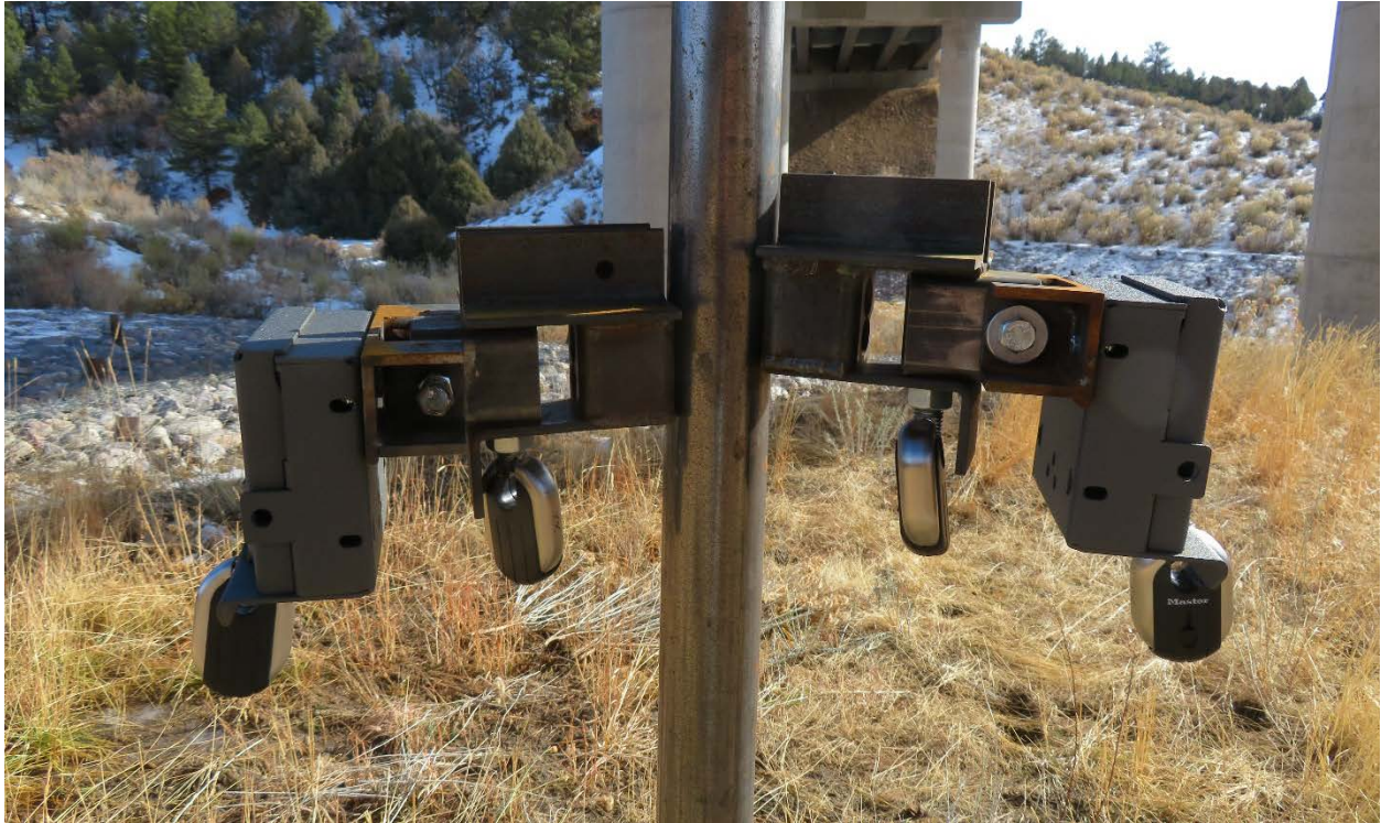
Figure 17. Pole A installation, looking east.
