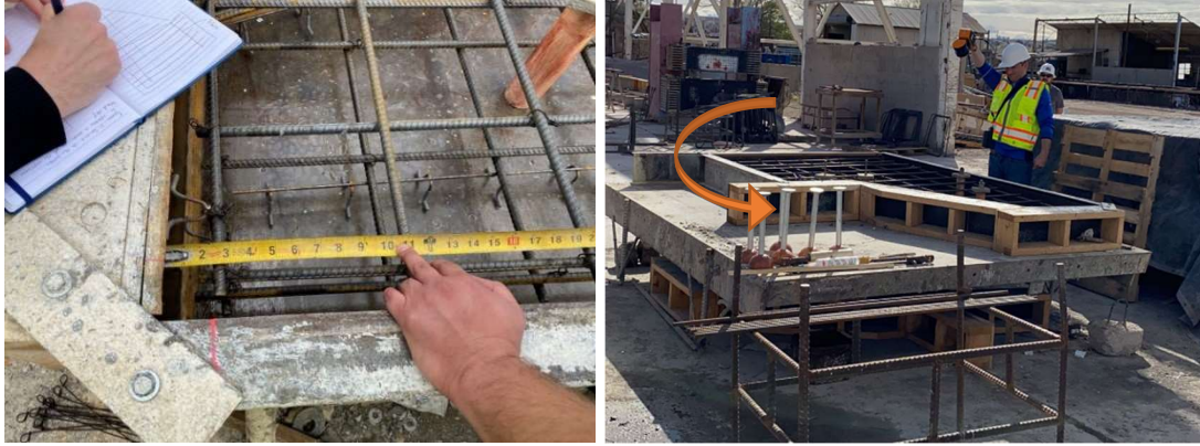
Figure 8. Data Collection. Left: Measurement by tape; Right: Measurement by LIDAR scanner.
