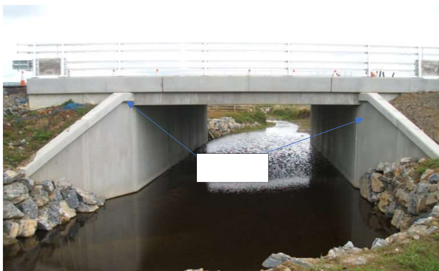
Figure 6. A constructed bridge with cantilevered flared wingwalls.
