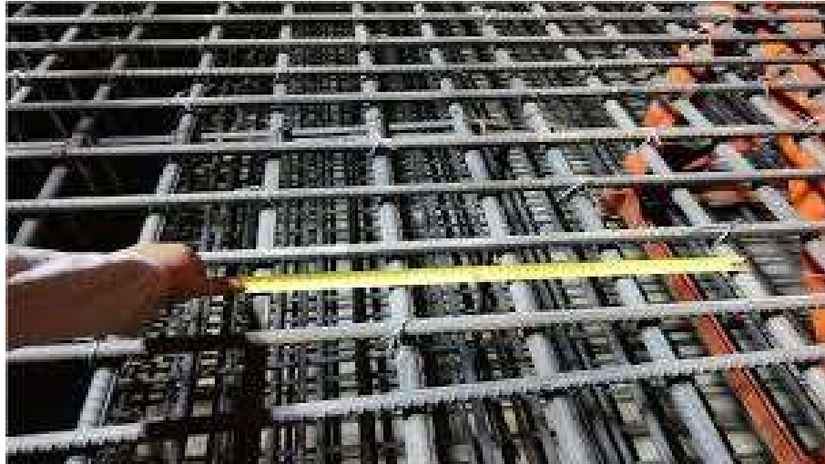
Figure 3. Bridge reinforcement placement inspection during construction.
