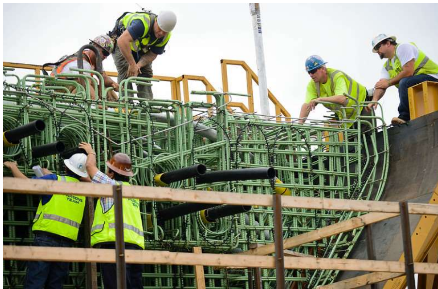
Figure 2. Bridge reinforcement during construction.
