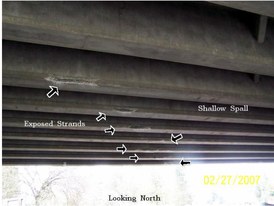
(c) Comparison with the observation from the real scenario – spallation of front faces at the bottom of girders
