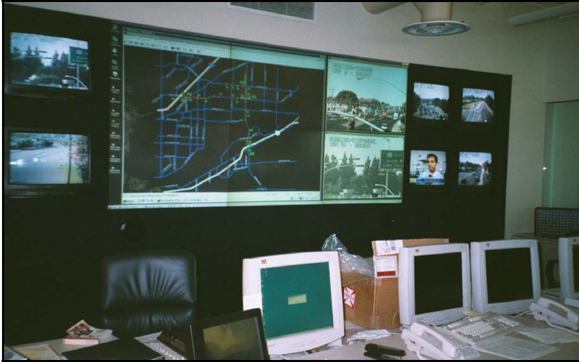
Figure 1-4. Sacramento County Traffic Operations Center.
