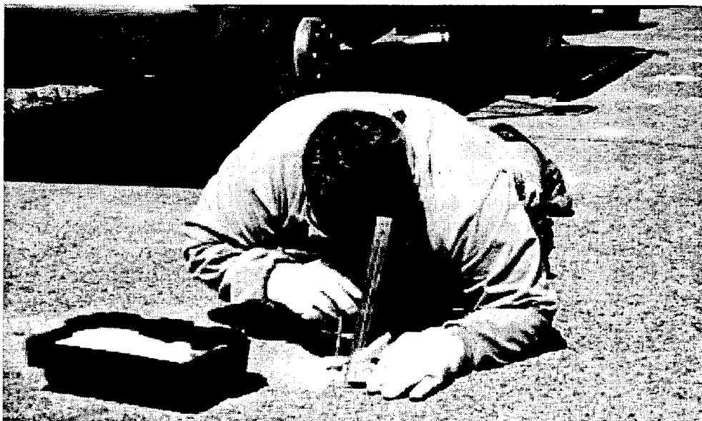
Figure 28: Installing Magnets
