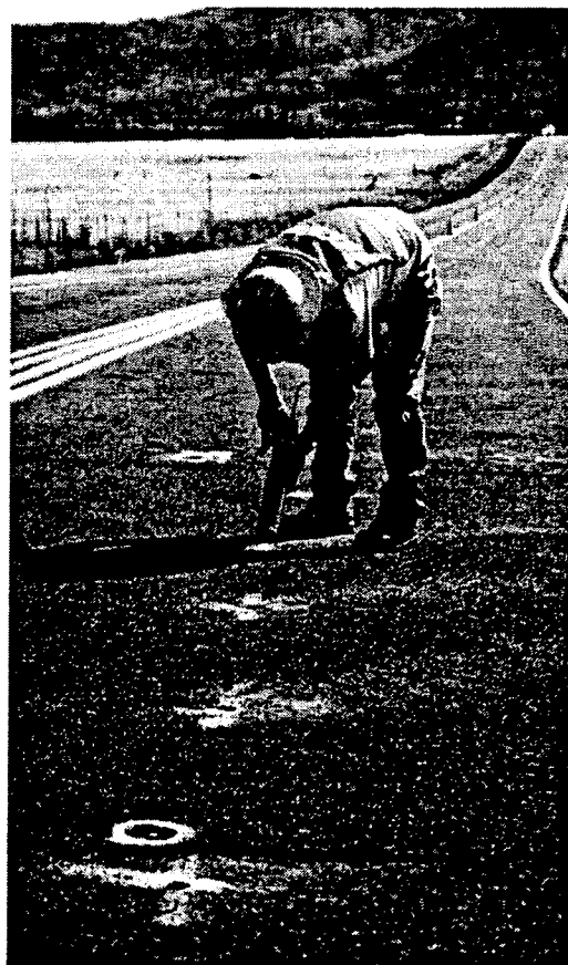
Figure 26: Setting and Sealing the PATH Magnets
