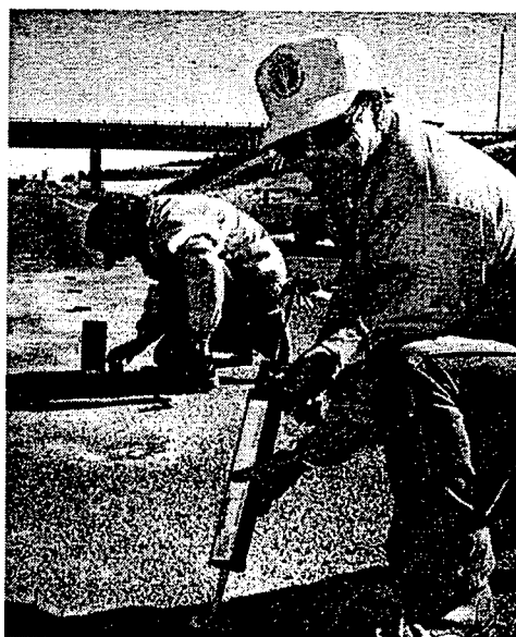
Figure 14: Installing and Sealing Test Magnets on I-40
