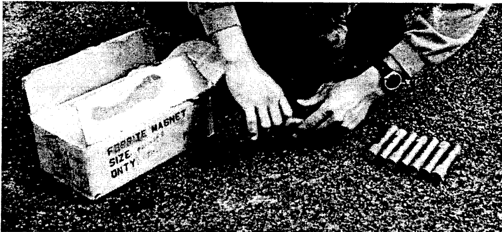
Figure 10: California PATH Discrete Magnetic Markers
