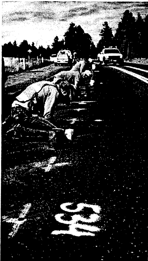
Figure 26: Setting and Sealing the PATH Magnets
