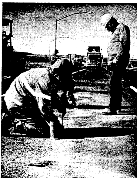
Figure 14: Installing and Sealing Test Magnets on I-40
