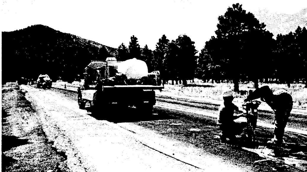
Figure 25: Four Two-man Crews on the Drill Line
