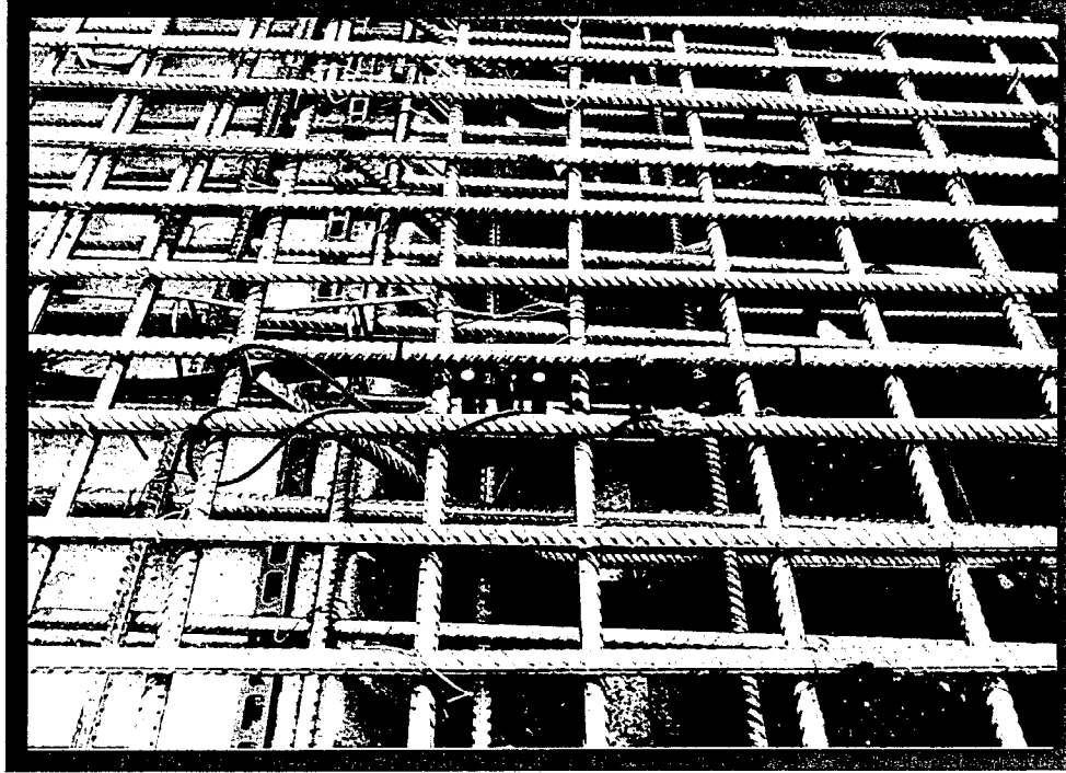
Garden State Parkway at State Rt. 80 Duplex alloy 2205 rebars
