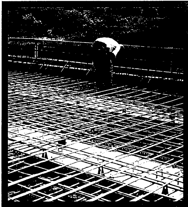
Figure 1. Stainless Steel Reinforcing Bar Installations
