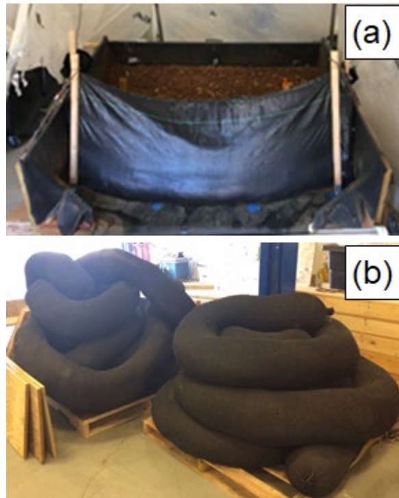
Figure 9. The sediment retention practices used in this study: (a) silt fence; (b) straw-filled and mulch-filled sediment tubes.
