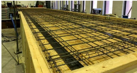
Figure 101. Deck reinforcement
