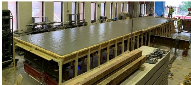
Figure 102. Deck concrete at completion of pour
