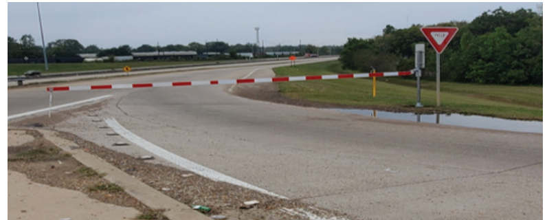
Figure 1. DOTD contraflow ramp closure gate
