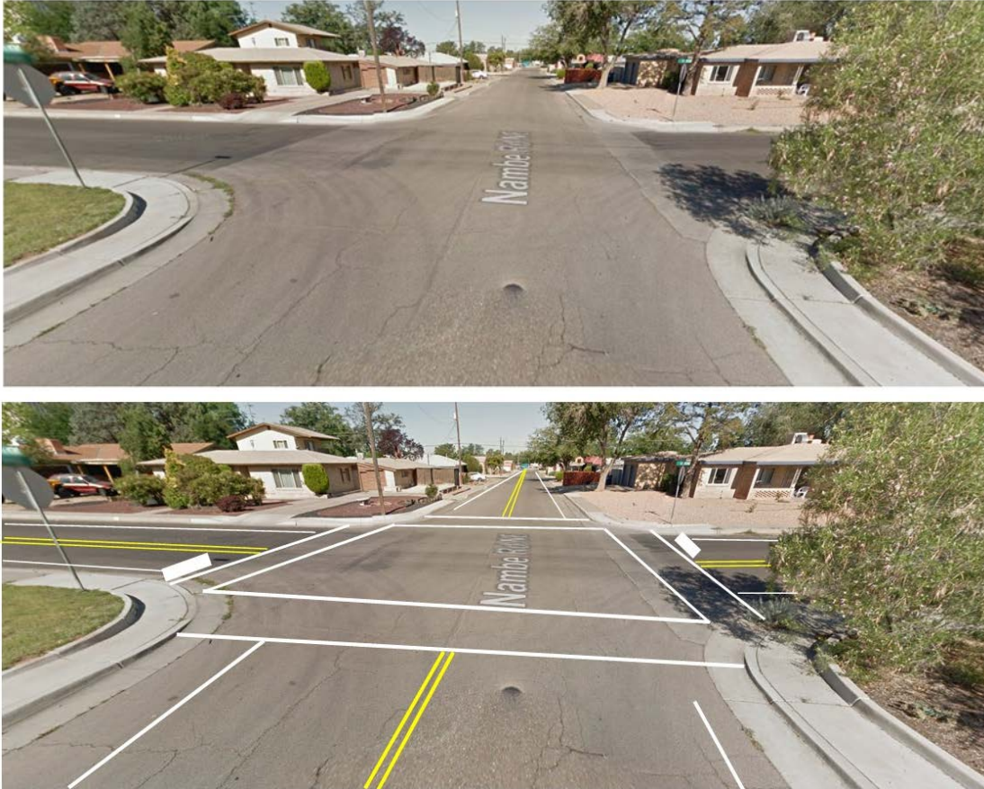
Figure 13. Pavement markings at an intersection (before and after).
