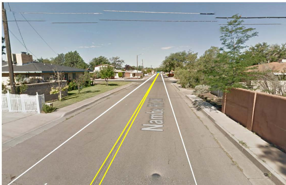
Figure 12. Pavement markings midblock (before and after).
