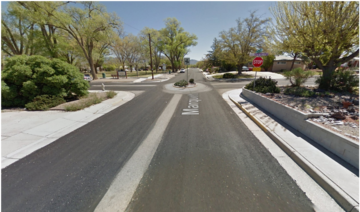
Figure 15. Traffic circle (before and after).
