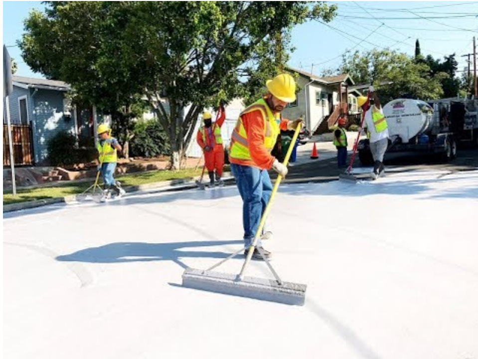
Figure 19. White asphalt sealant installation.
