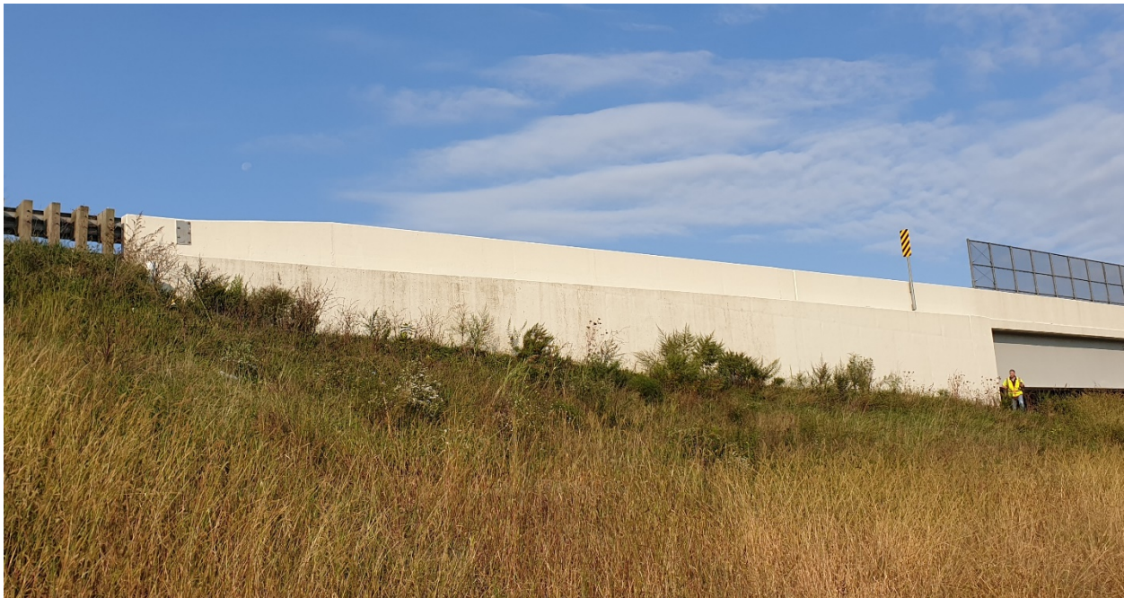
Figure 3.2 The Right Forward Abutment Wing Wall (Wall 3)
