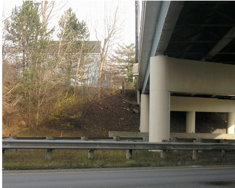
Photograph 3: Spill-through Slope at Forward Abutment
