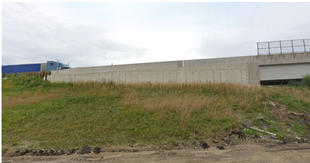
Figure 4.6 CUY-77-14.35 Wall 4 (Google Maps)
