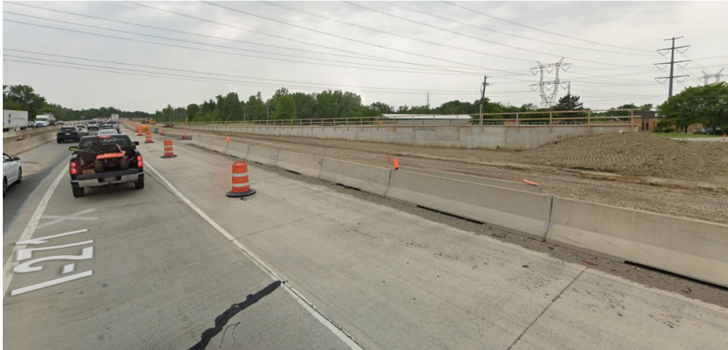
Figure 4.2 Picture of I-271 Wall (Google Maps)
