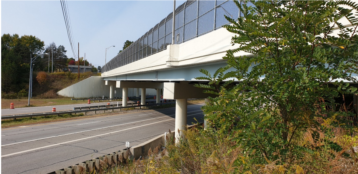
Figure 3.1 The MAH-680-0283 Bridge
