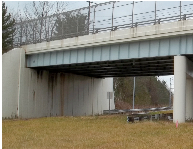
Photograph 2: Reinforced Concrete Retaining Wall at Rear Abutment
