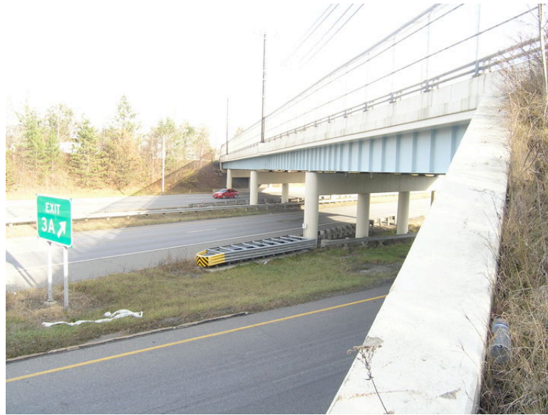
Photograph 1: Existing Four-Span Structure Looking East
