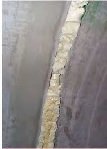
Internal Chemical Grouted Joint (RCP)
