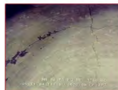
Typical Locations for Longitudinal Cracking can be Found in the Crown and Invert.
