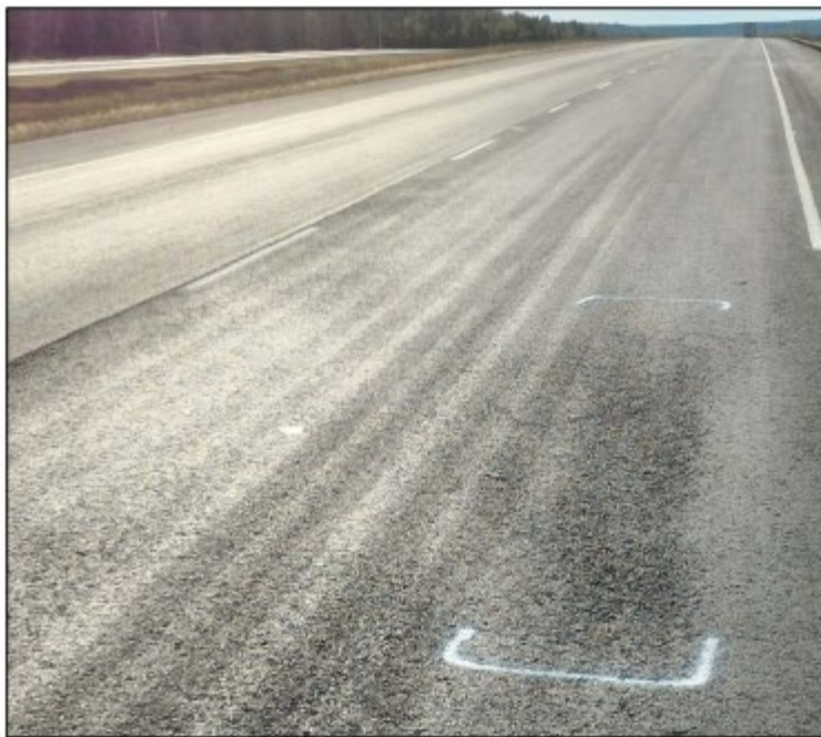
Photograph 8 - Moderate (bordering on Severe) Segregation
