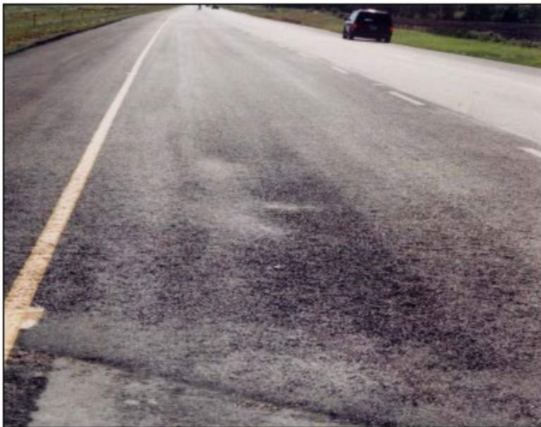
Photograph 10 - Severe Segregation
