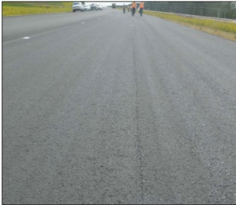
Photograph 13 - Centre-of-Paver Streak
