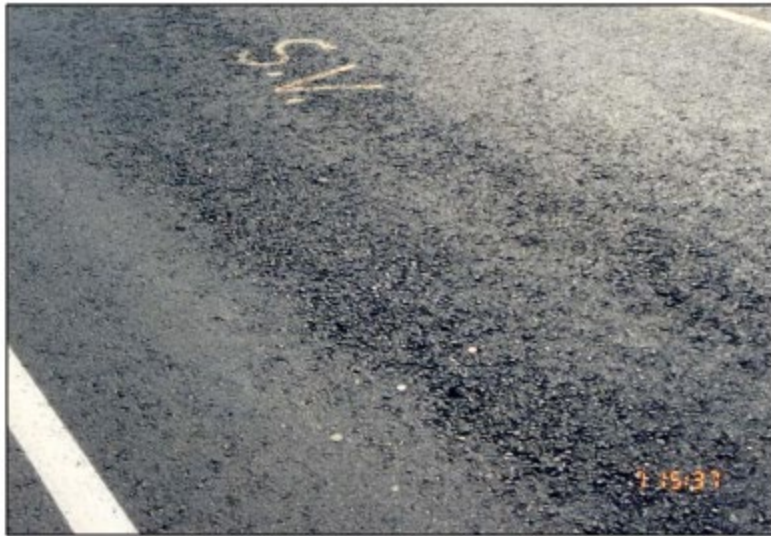
Photograph 11 - Severe Segregation
