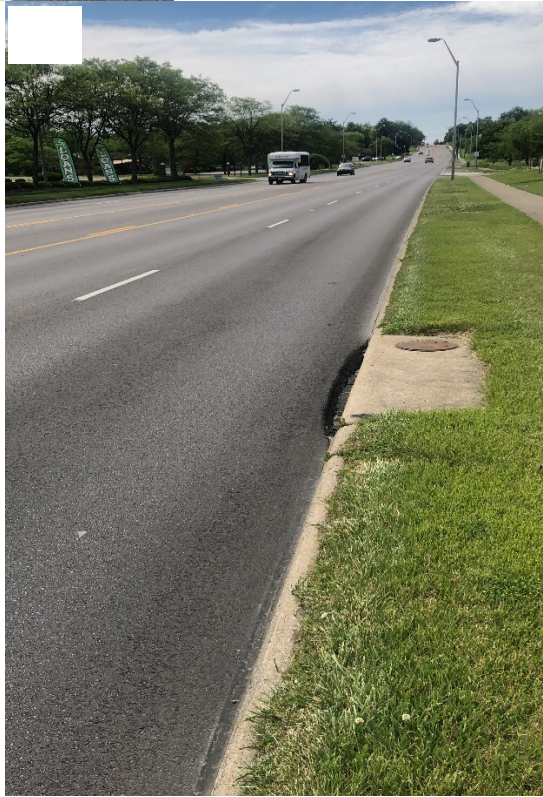
Figure B.17 Pictures Taken of city of Columbus Test Sections after Six Months of Construction: a) City of Kettering- PG 64-22 + Fiber A section, b) City of Kettering- PG 64-22 + Fiber B section, and c) City of Kettering- PG 70-22M section.
