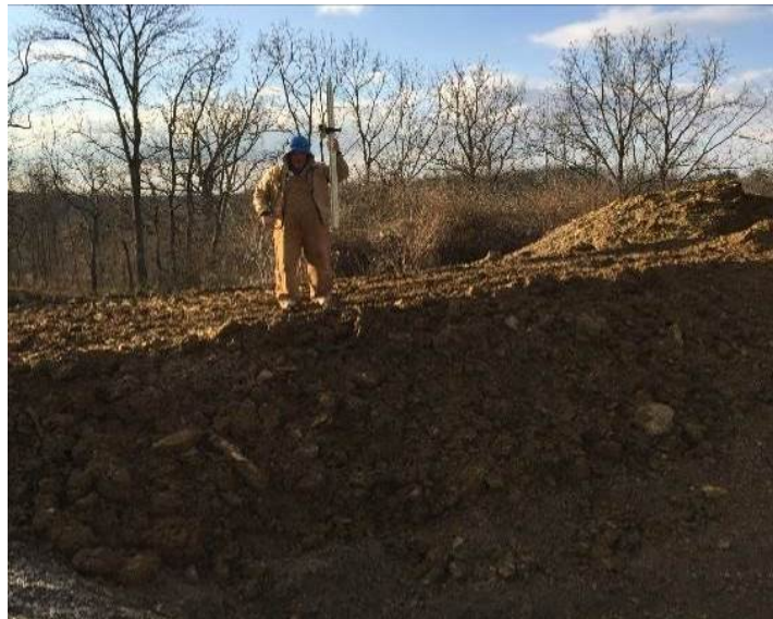
Figure 17. Rod being held during backfill height measurement by laser plane.
