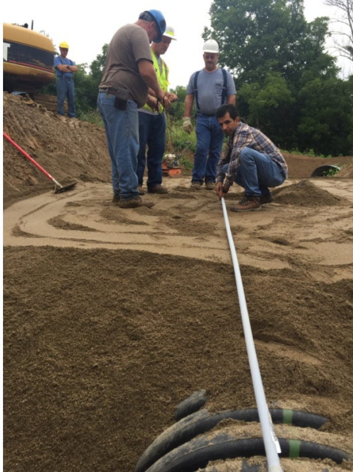
Figure 31. Positioning accelerometers above crown of Pipe 2.
