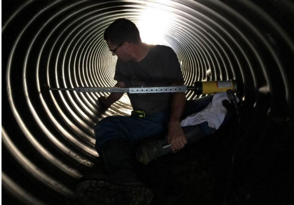
Figure 37. A hydraulic jack was used to measure soil resistance before and after re-rounding.
