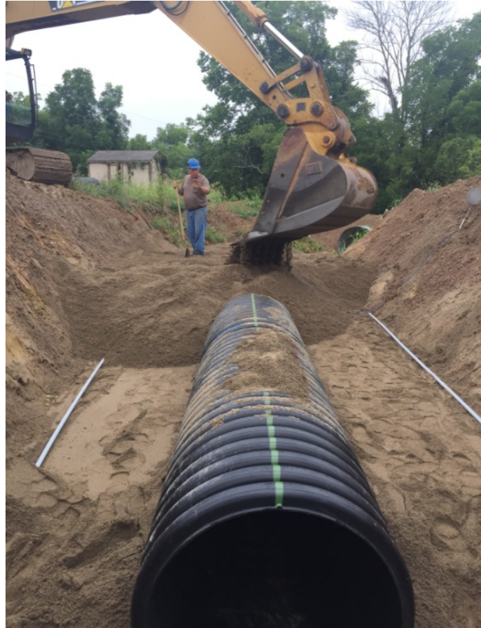
Figure 30. Placing ODOT Type 2 backfill sand around Pipe 2.
