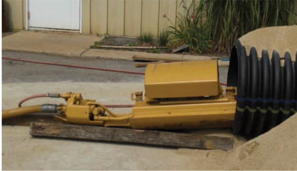
Figure 1. Pipe re-rounding device at pipe entrance [ADS, 2009].
