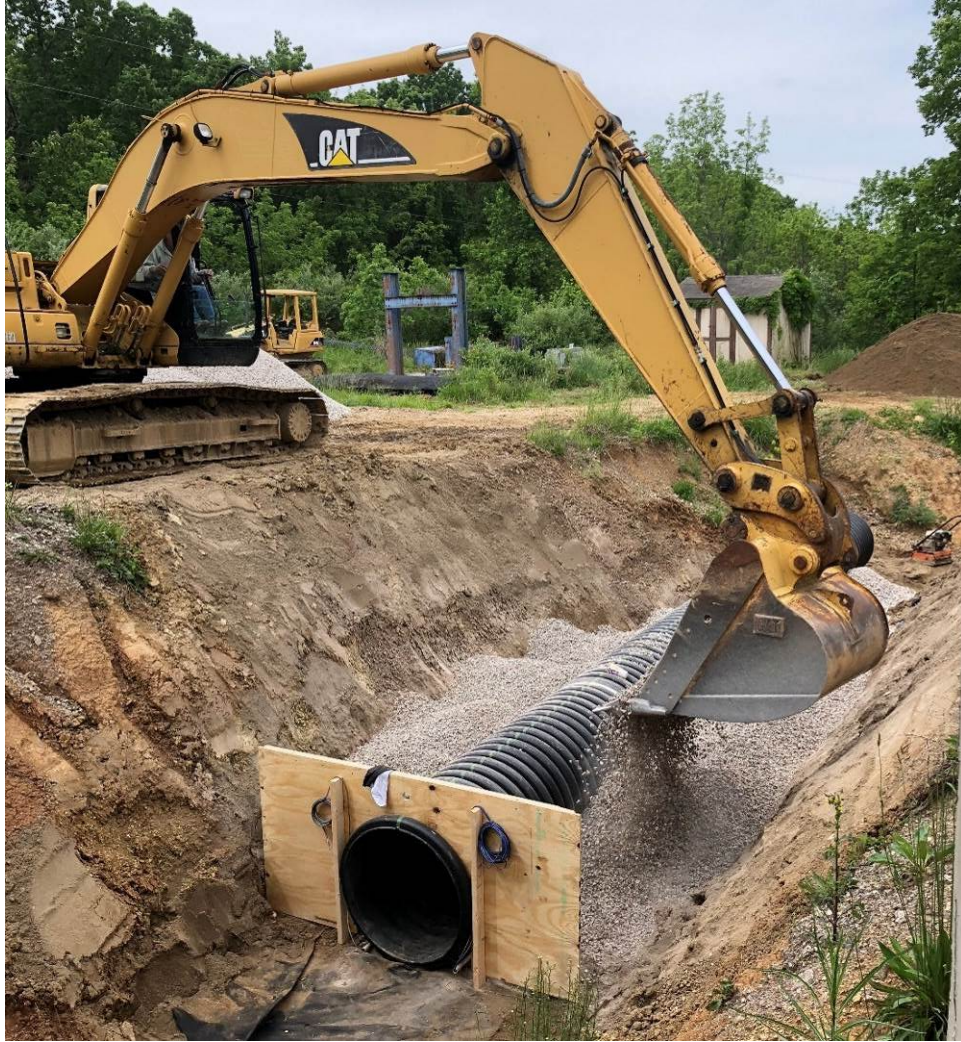
Figure 38. Placement of Structural Backfill Type 3 on Test Pipe 3.
