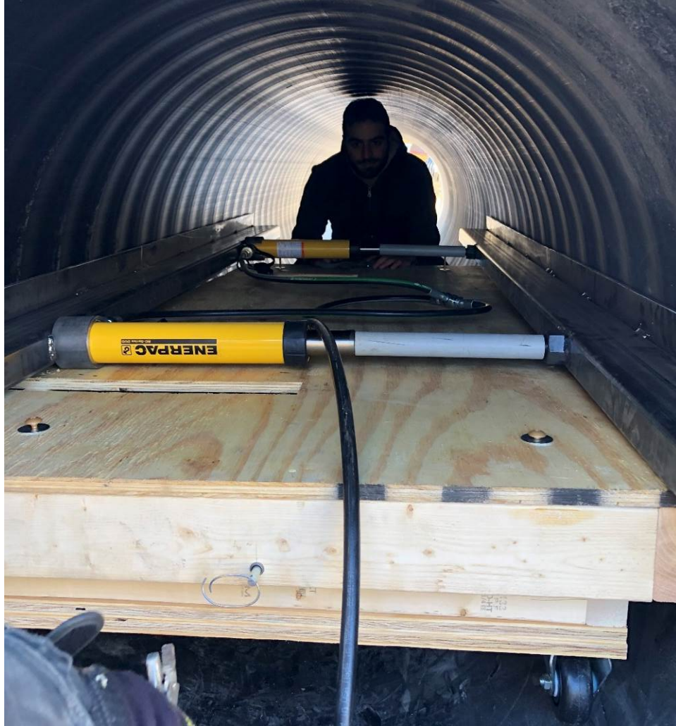
Figure 43. Actuated deflection device and delivery system showing the deformed pipe section.
