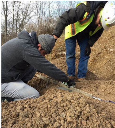
Figure 24. Positioning pressure cell above the pipe crown.
