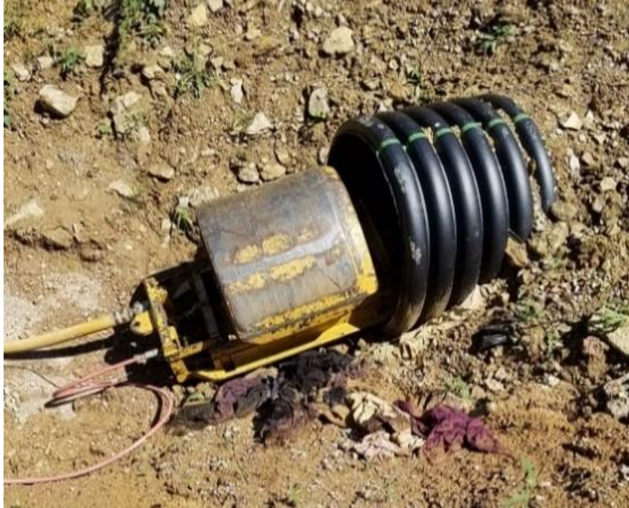
Figure 27. Re-rounder positioned at entrance to the pipe at start of re-rounding.
