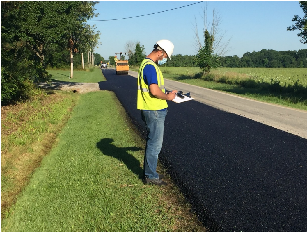
Figure B.4: Placement of Asphalt Mixture at the Medina County Test Site.
