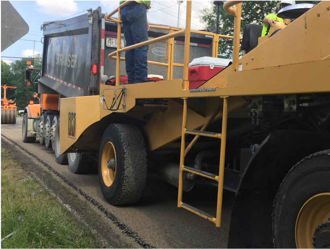
Figure A.6: Choking with No. 9 Limestone at the Franklin County Test Site.
