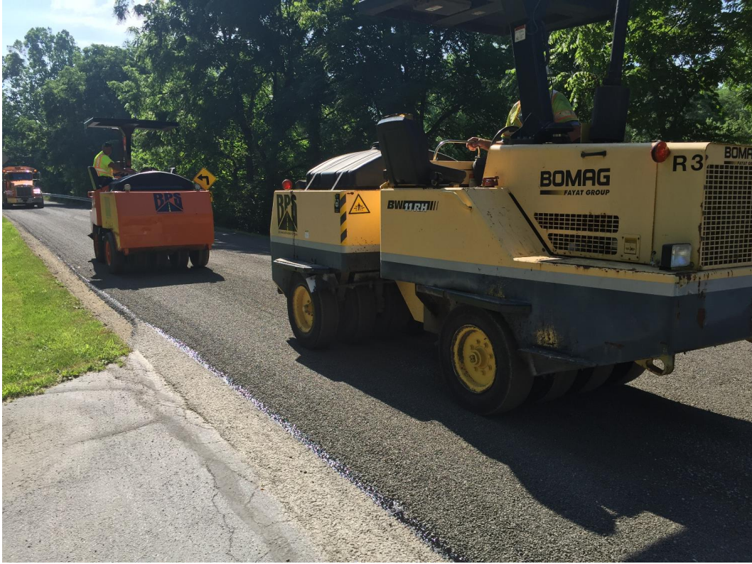
Figure A.7: Chip Sealing at the Franklin County Test Site (Continued).
