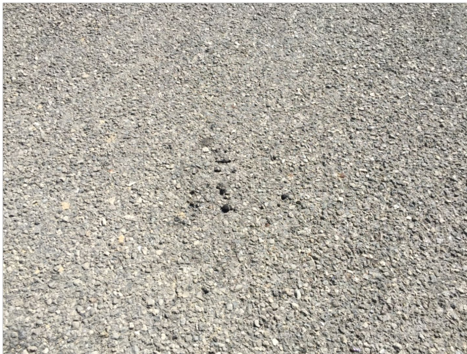
Figure D.3: Limited Aggregate Loss from the Chip Seal Layer at the Franklin County Test Site.
