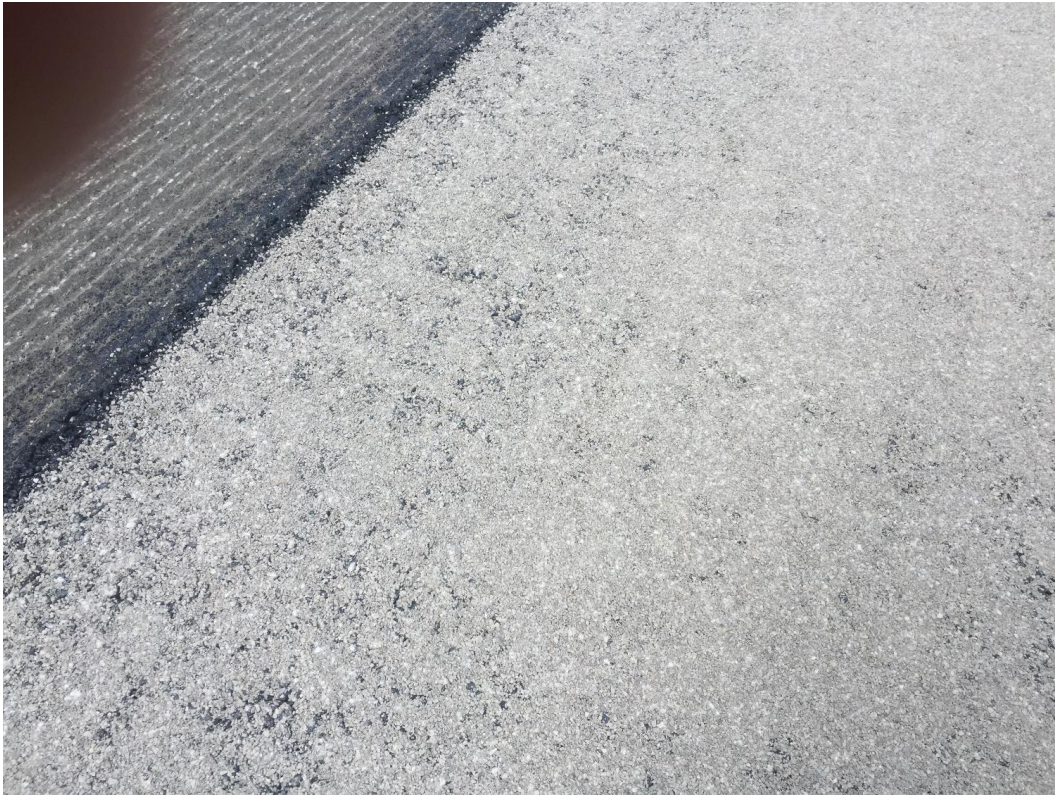
Figure A.6: Choking with No. 9 Limestone at the Franklin County Test Site (Continued).
