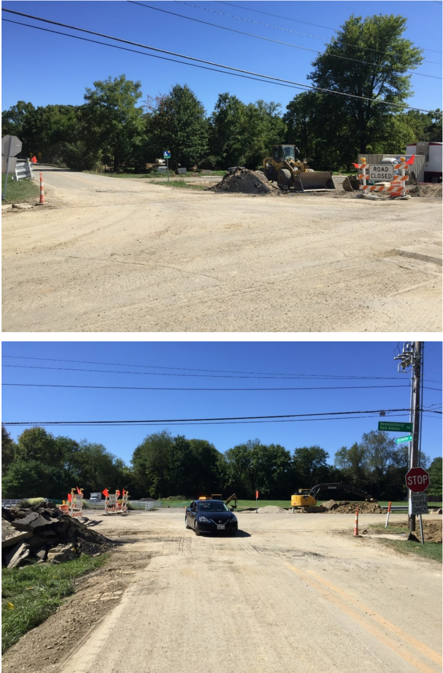
Figure D.1: Effect of Nearby Construction on the Southern Part of the Franklin County Test Site.
