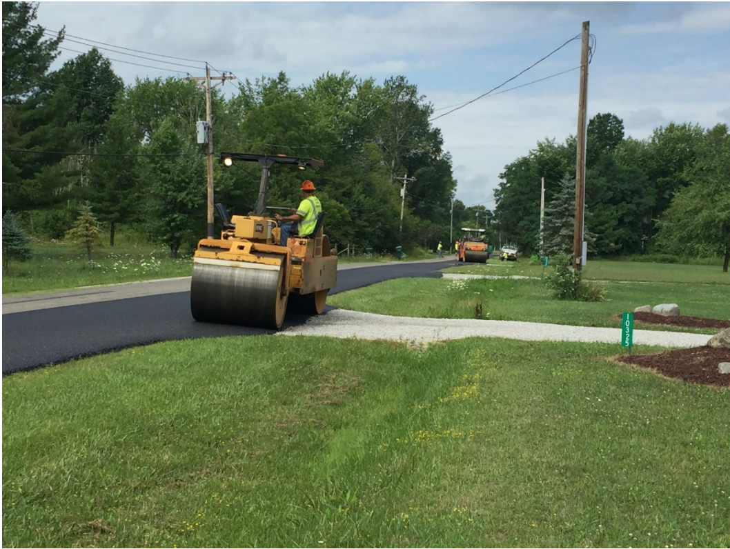
Figure B.5: Compaction of Asphalt Mixture at the Medina County Test Site.
