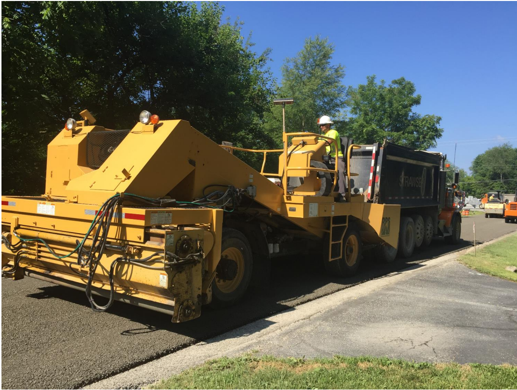
Figure A.7: Chip Sealing at the Franklin County Test Site.
