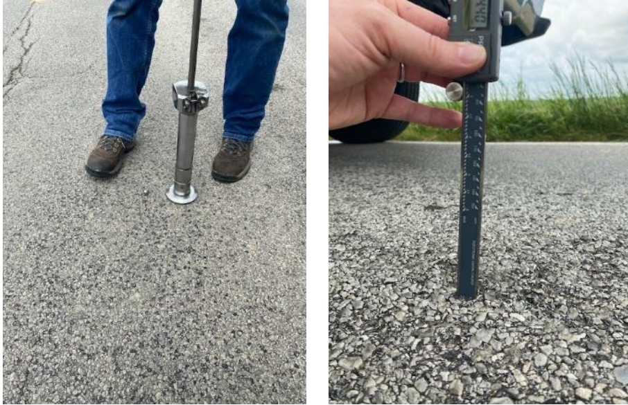
Figure 8-6 Ball Penetration Test on Chippewa Rd., Wayne County, OH
