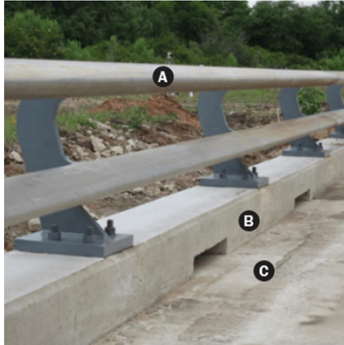
Figure 5.3 Bridge Curb Opening: (a) Steel Bridge Rail (b) Concrete Curb (C) Bridge Slab (TxDOT, 2021)
