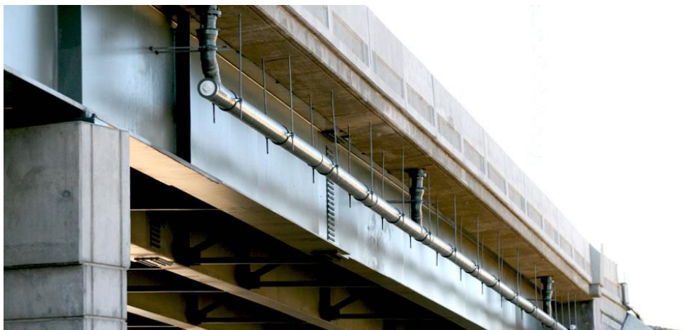
Figure 2.9 Bridge Deck Drainage Pipes (Hennegan & Associates, 2020)
