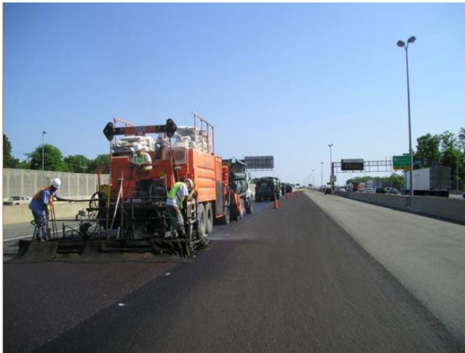
Figure 27. Photo. Slurry Seal Operation (Source: Bill Evans, Ergon)
