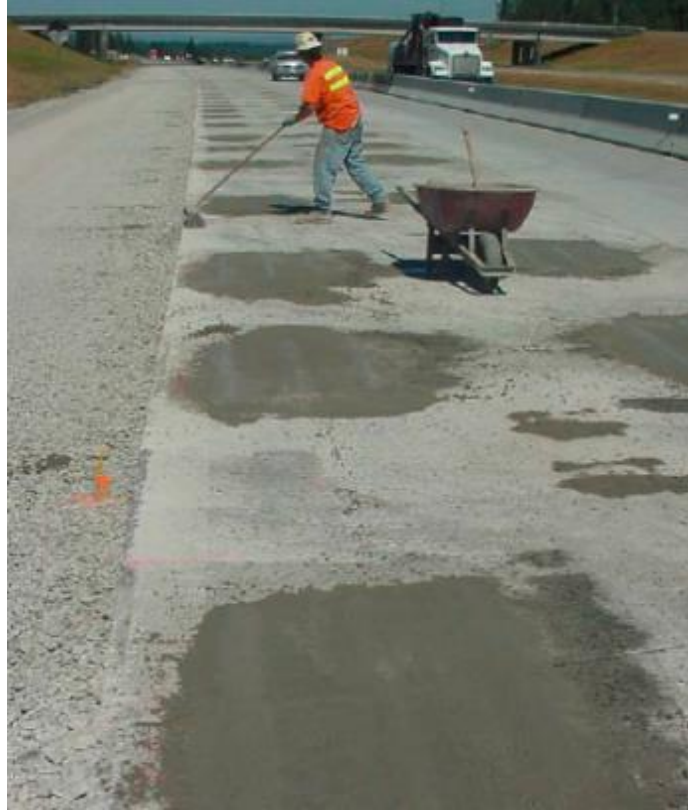
Figure 91. Photo. Completed placement of patching material (Bischoff et al., 2002)
