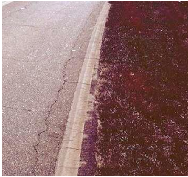
Level 1 – tight, hairline cracks
