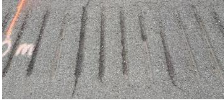
Figure 198. Photo. Site 1 Wet Aggregate in Rumble Strip
