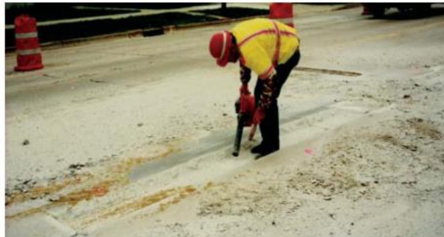
Figure 74. Photo. Using a Leaf Blower for Final Removal of Any Contaminants
