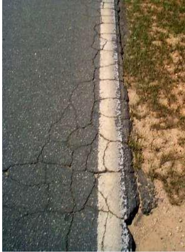
Level 2 – crack widths greater than 1/4 inch, double cracking, tight “alligator” cracking
