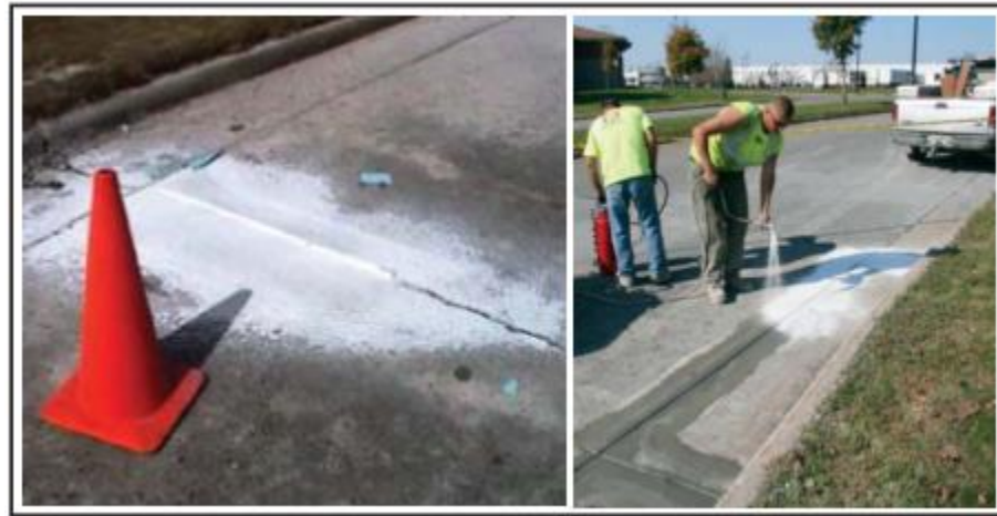
Figure 77. Photo. Curing of Repair Material (Frentress et al., 2012)
