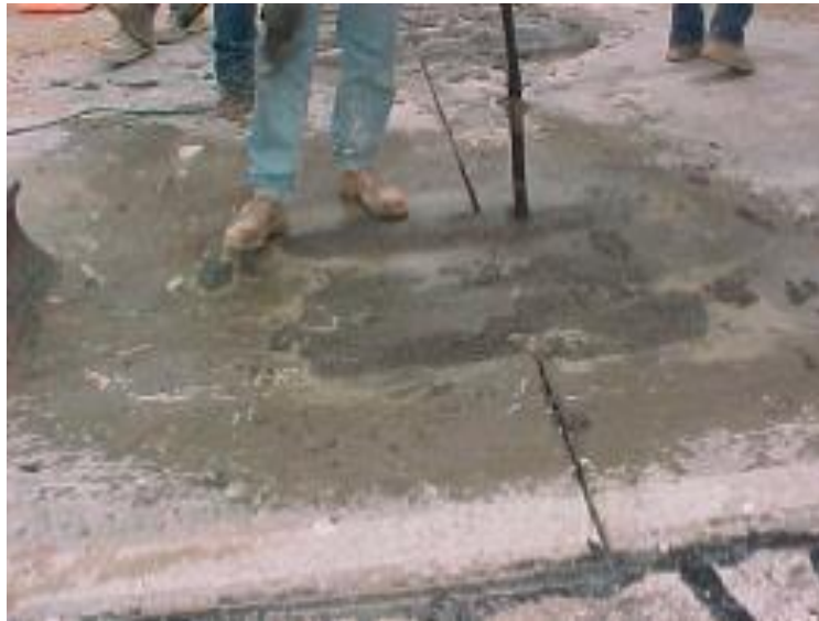
Figure 90. Photo. Patching material consolidation (Bischoff et al., 2002)
