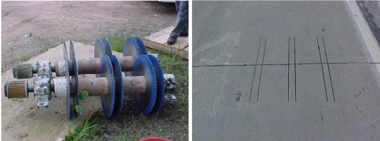
Figure 84. Photo. Cutting Slots (Bischoff et al., 2002)
