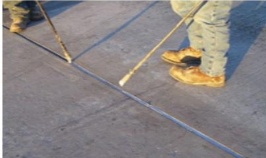
Figure 102. Photo. Sealant Placement at left followed by tooling operation at right (CP Tech Center)
