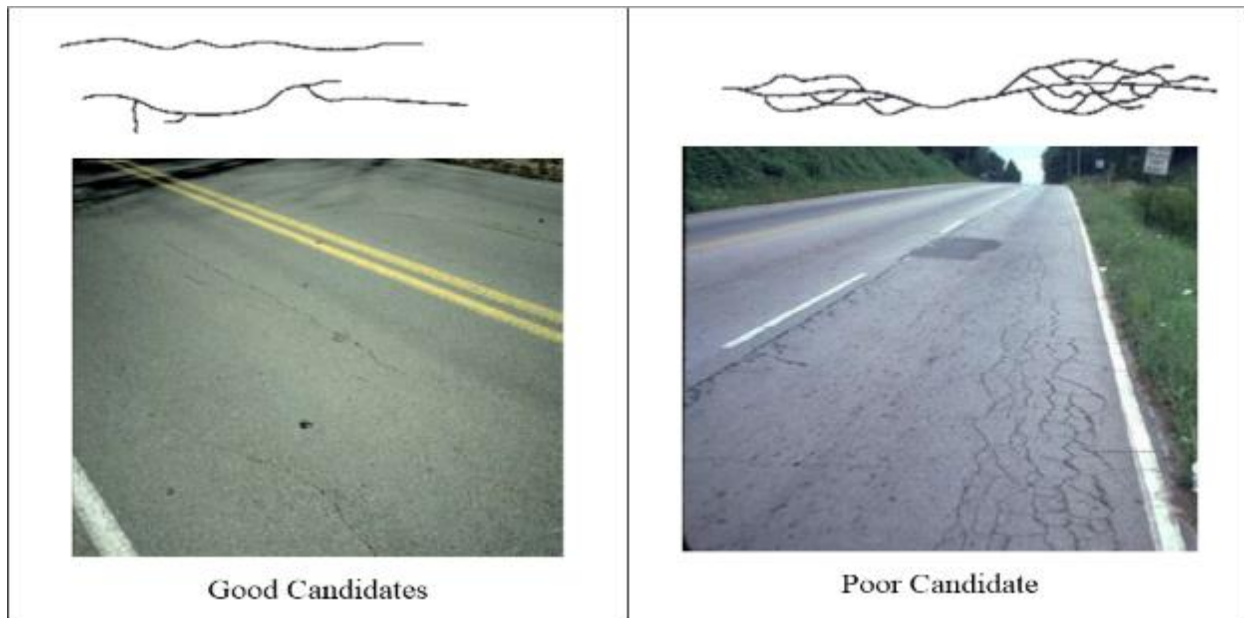
Figure 6. Photo. Cracking Characteristics of Good and Poor Candidates (Decker, 2014; GDOT, 2007)
