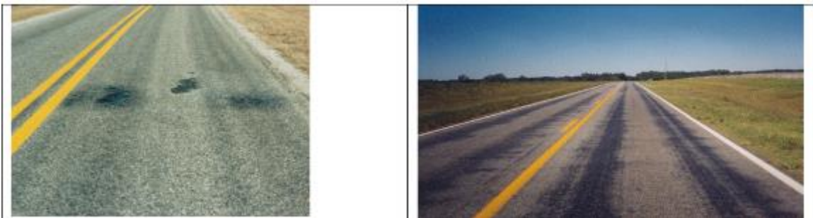
Figure 22. Photo. Bleeding Joint and Bleeding Wheel Paths
