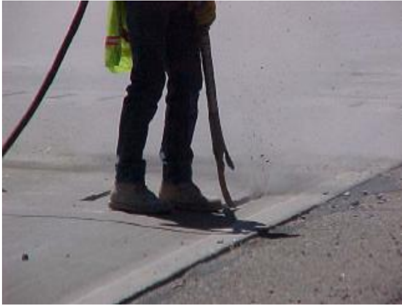
Figure 85. Photo. Compressed Air Used to Blow Any Debris Out of the Slots
