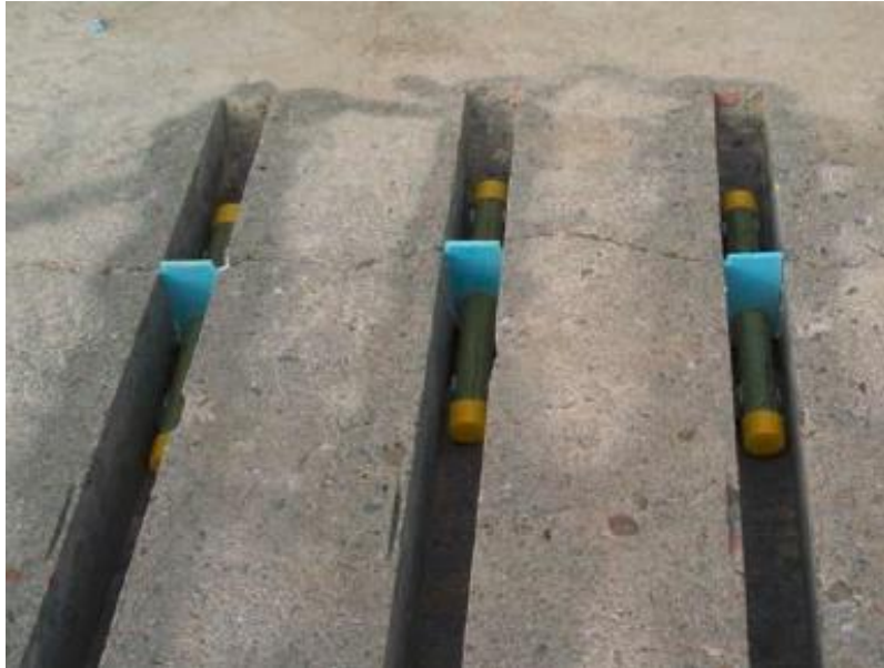
Figure 87. Photo. Dowel bars after placement
