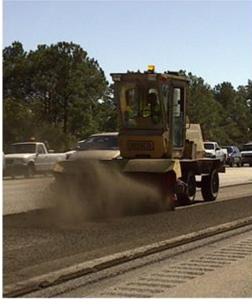
Figure 36. Photo. Cleaning a Micro-milled Surface
