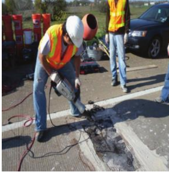
Figure 69. Photo. Removal Concrete with a Jackhammer (Jungheum, 2012)
