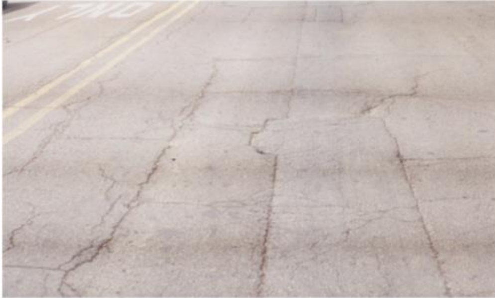
Figure 45. Photo. Pavement distress suitable for HIR (NCAT, 2011)
