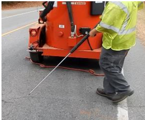
(a) Crack Clean (clean first)
