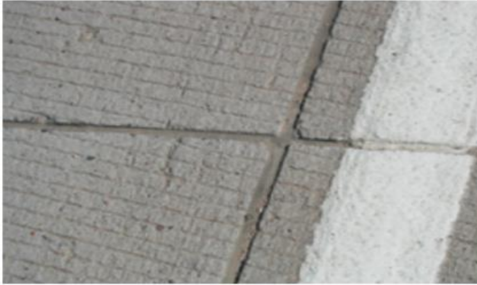
Figure 100. Photo. Joint Sealed with Silicone Material (CP Tech Center)
