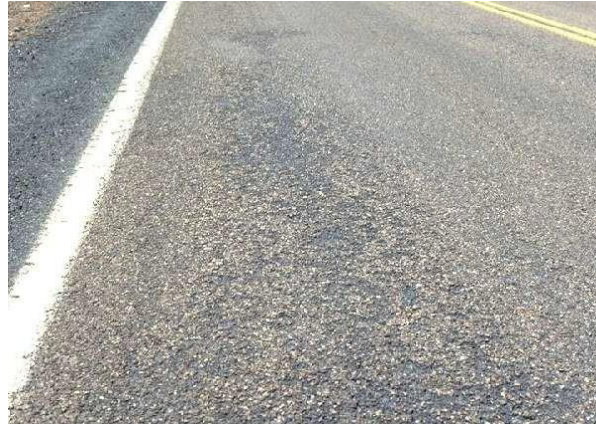
Level 2 – loss of most surface
