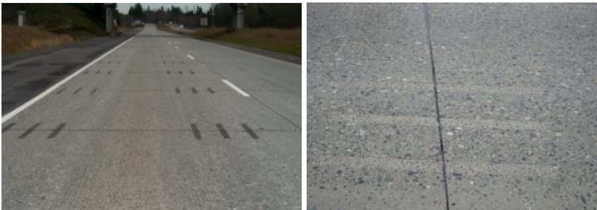
Figure 82. Photo. Completion of Dowel Bar Retrofit (Pavement Interactive, 2014)
