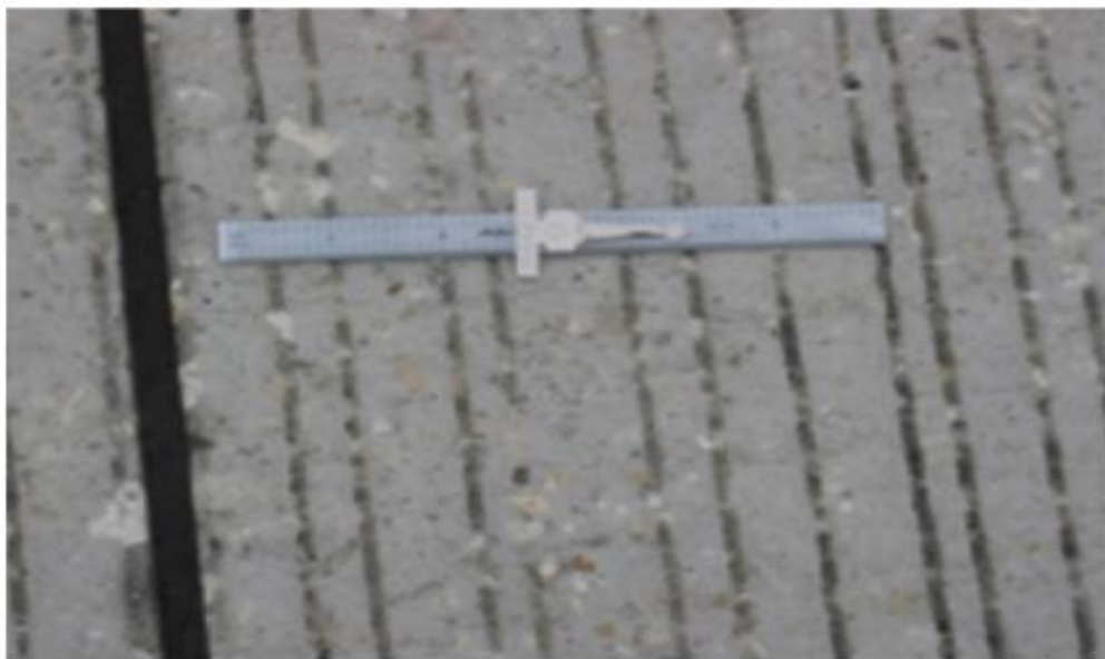
Figure 99. Photo. Joint Sealed with Hot-applied Thermoplastic Material (CP Tech Center)
