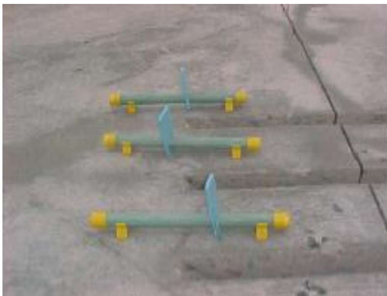
Figure 86. Photo. Each dowel bar after preparation fitted with two end caps, two chairs, and a foam board (Bischoff et al.,2002)
