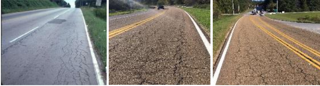
Figure 25. Photo. Characteristics of Poor Candidates for Slurry Seal (GDOT, 2007)
