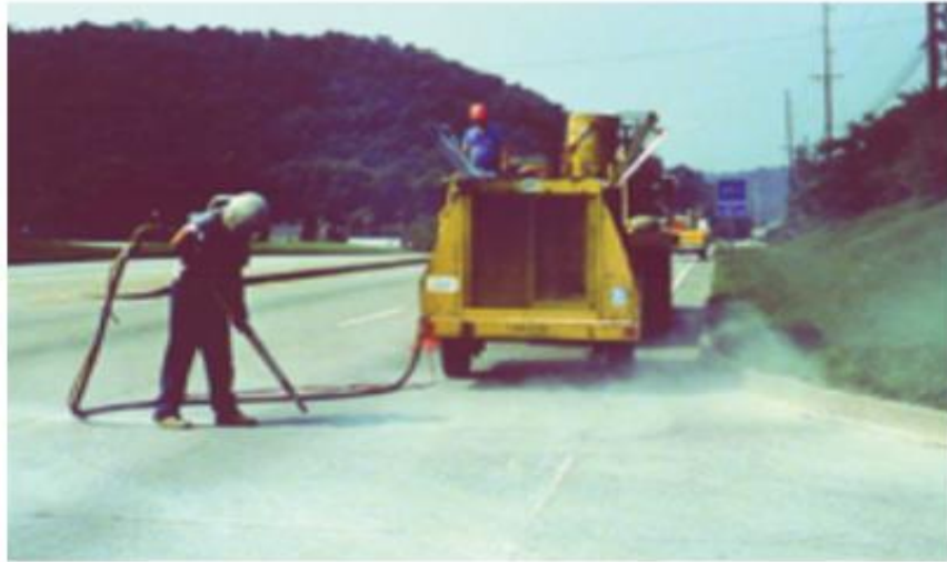
Figure 104. Photo. Sandblasting along a transverse joint (CP Tech Center)
