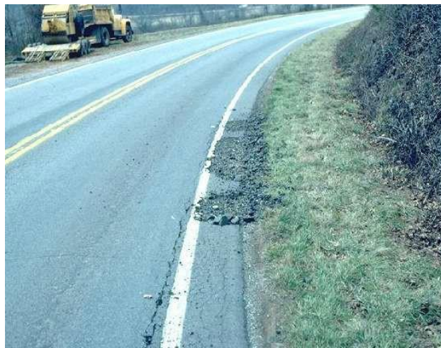
Level 3 – severe “alligator” cracking at edge, popouts, edge break off
