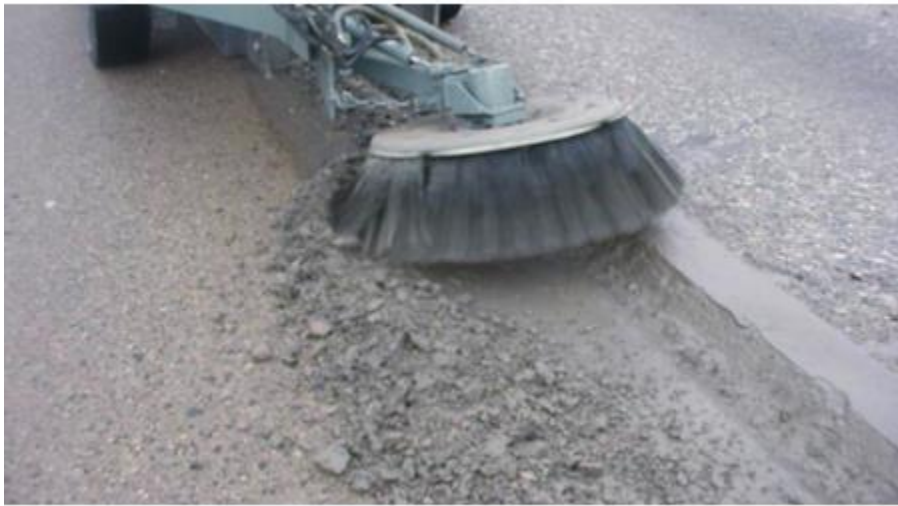
Figure 71. Photo. Sweeping Loose Material (Frentress et al., 2012)
