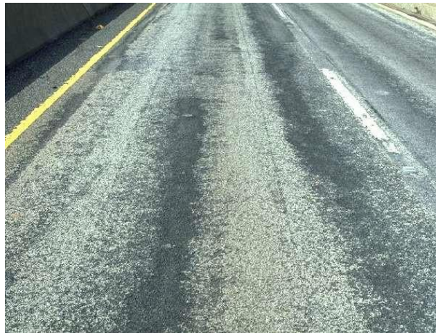
Level 3 – loss of substantial portion of surface layer ( >1/2 depth)
