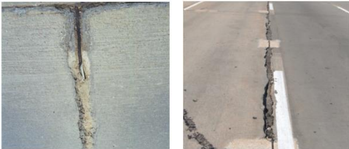
Figure 65. Photo. Spot repair (Left) and Long Joint/Crack Repair (right) (Daniel, 2011)
