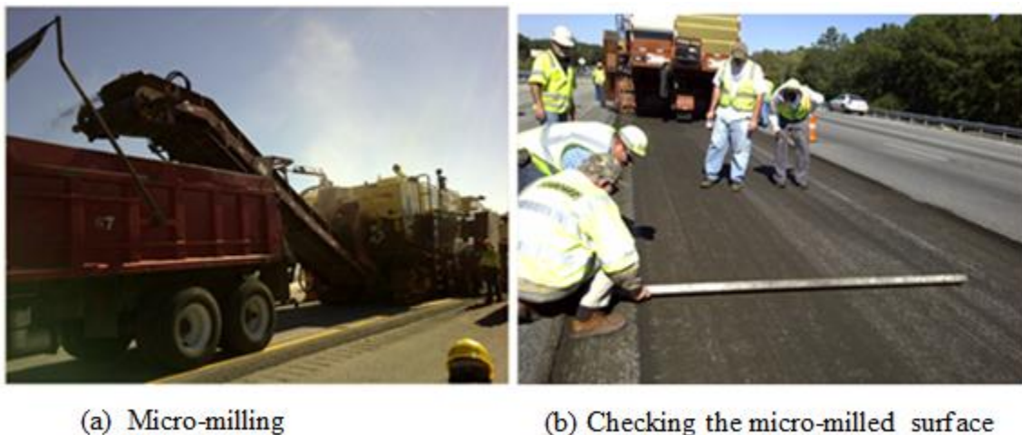
Figure 35. Photo. Micro-milling Operation
