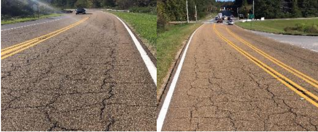
Figure 32. Photo. Bad Candidates for Thin Overlay
