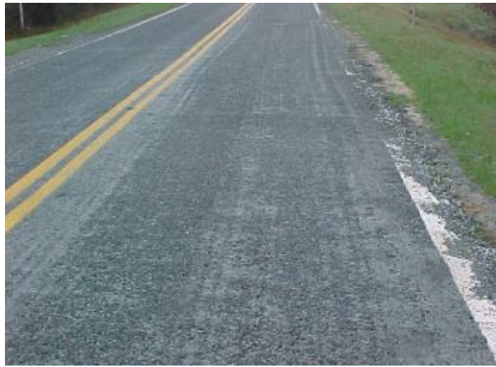
Figure 23. Photo. Streaking/Raveling
