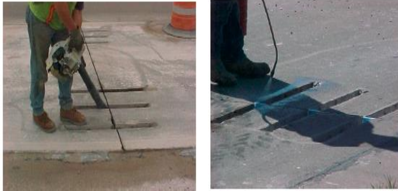
Figure 89. Photo. Slot preparation before patching (Bischoff et al., 2002)
