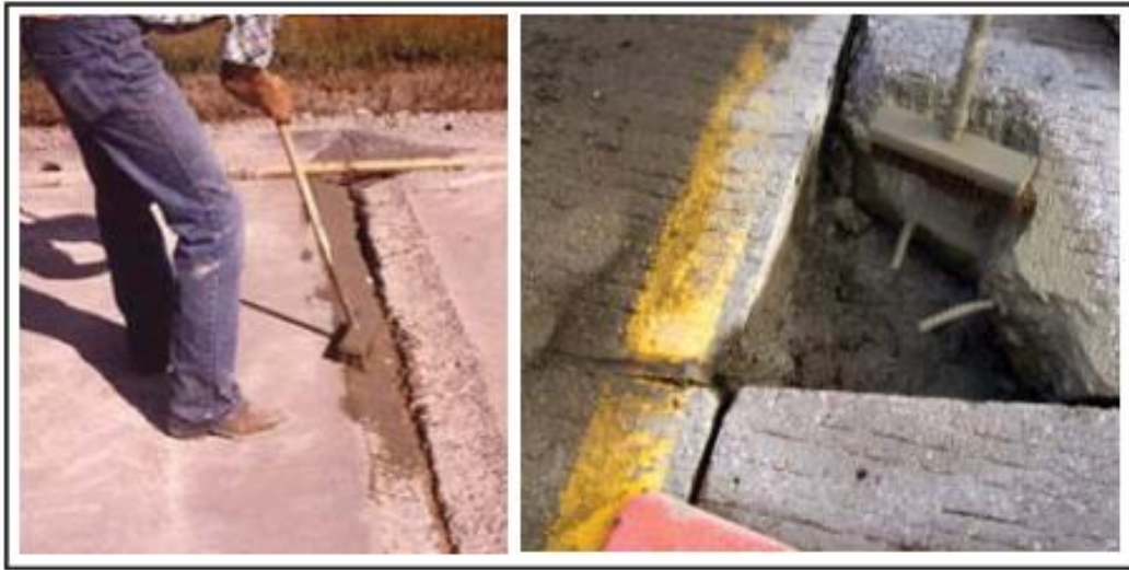
Figure 75. Photo. Placement of Cement Grout as Bonding Agent (Frentress et al., 2012)
