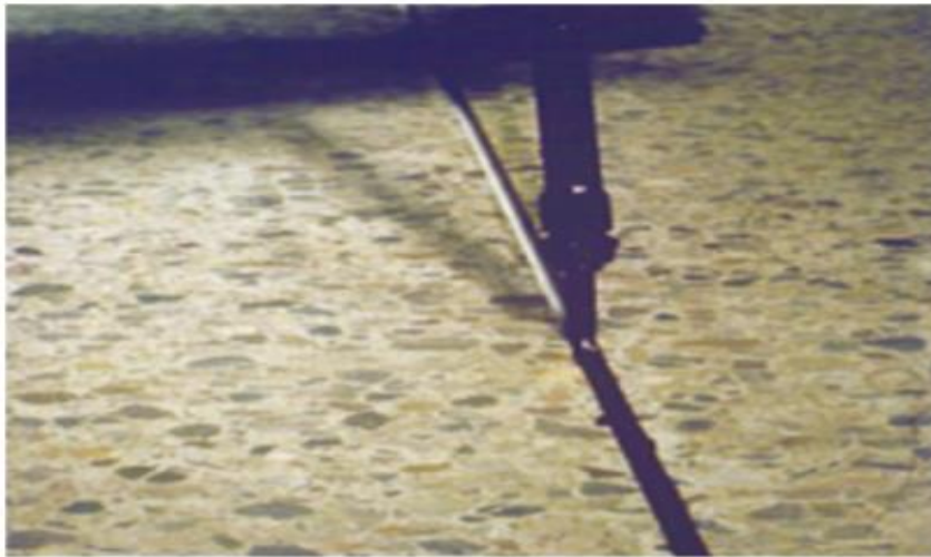
Figure 101. Photo. Installation of hot-applied joint sealant
