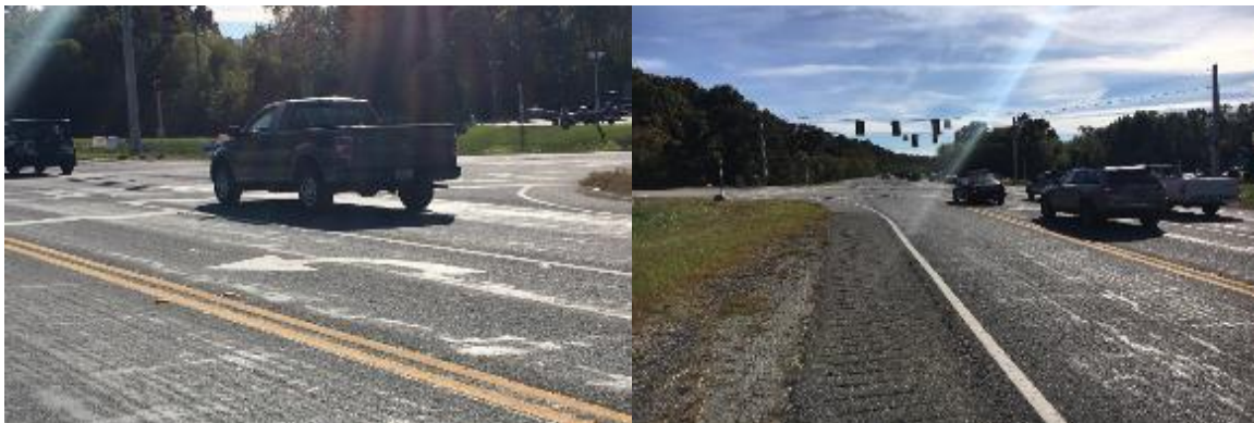
Figure 15. Photo. Poor Candidates for Chip Seal
