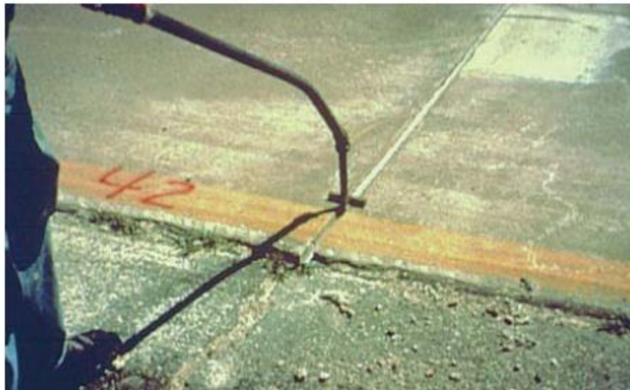
Figure 78. Photo. Joint sealing (Frentress et al., 2012)
