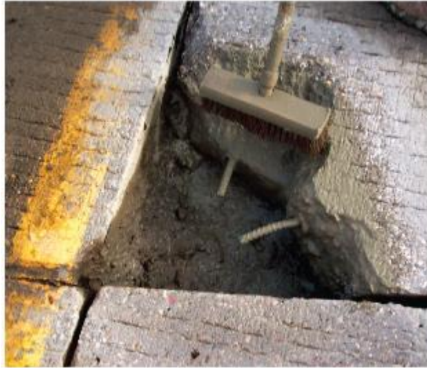
Figure 66. Photo. Deteriorated Pavement Corner (Daniel, 2011)
