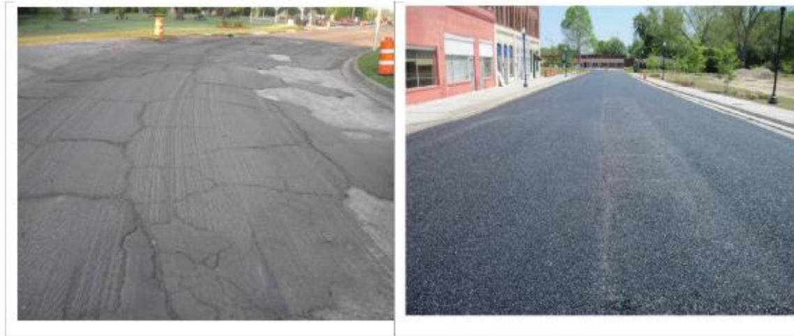
Figure 41. Photo. OGI Project (a) Before OGI and (b) After OGI (GDOT)
