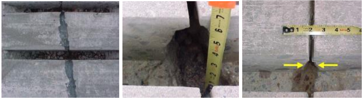
Figure 92. Photo. Potential pavement issues for dowel bar retrofit (Bischoff et al., 2002)
