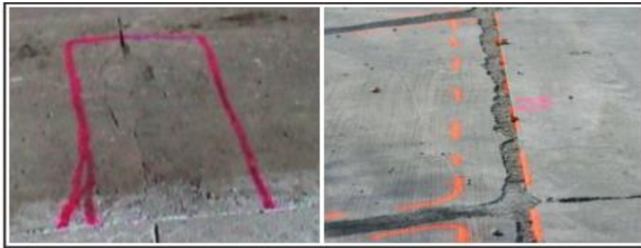
Figure 68. Photo. Deteriorated Pavement Marked for Sawing (Frentress et al., 2012)
