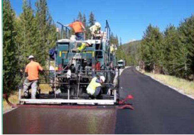
Figure 29. Photo. Micro-surfacing Operation (NCP, 2017)
