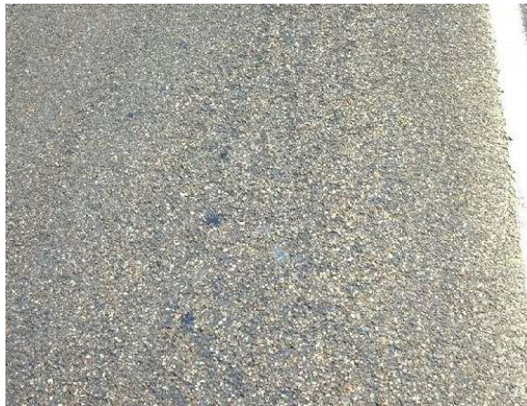
Level 1 – loss of substantial number of stones
