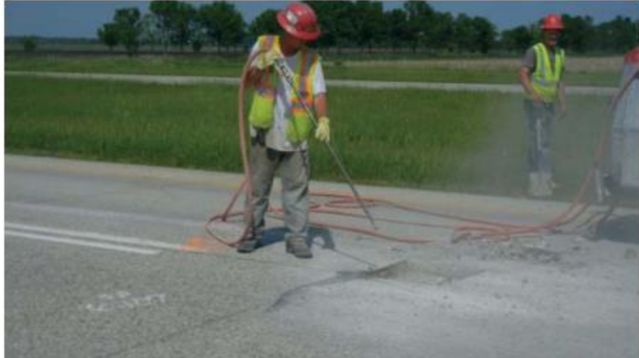
Figure 73. Photo. Air Blasting to Remove Loose Debris (Frentress et al., 2012)
