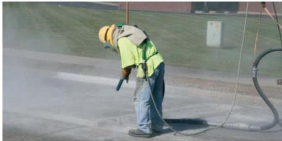
Figure 72. Photo. Sandblasting to Remove Loose Debris (Frentress et al., 2012)
