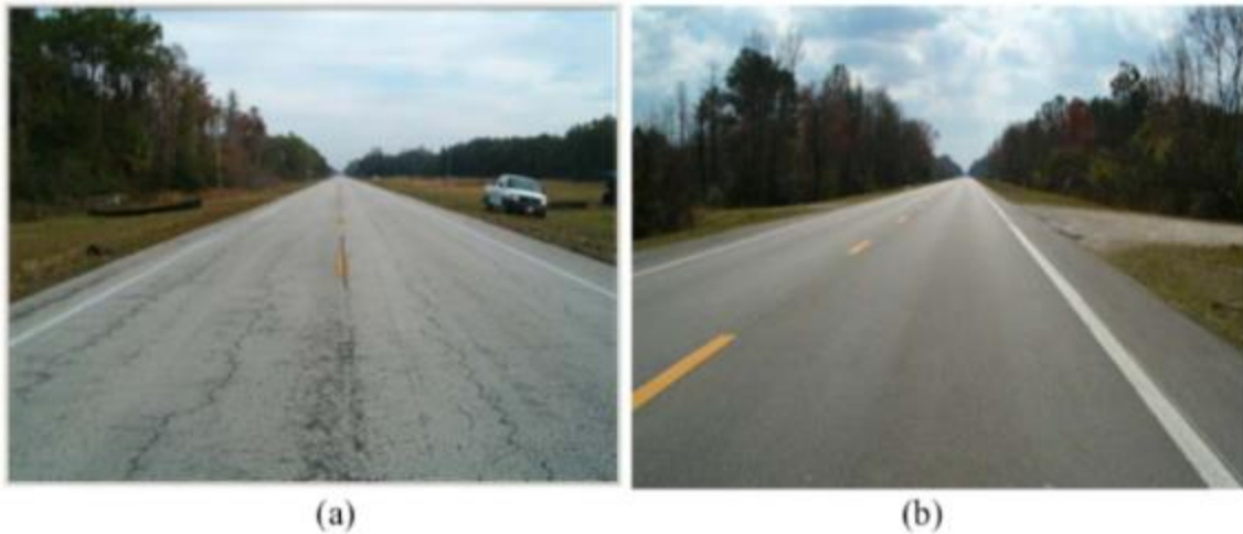
Figure 44. Photo. HIR Project (a) Before HIR and (b) 7 Years Later (NCAT, 2011)
