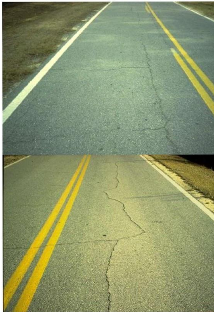
Examples of Level 1 Block/Transverse Cracking
