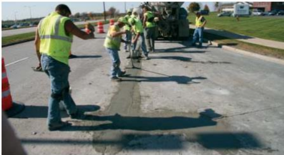
Figure 76. Photo. Placement of Repair Material (Frentress et al., 2012)
