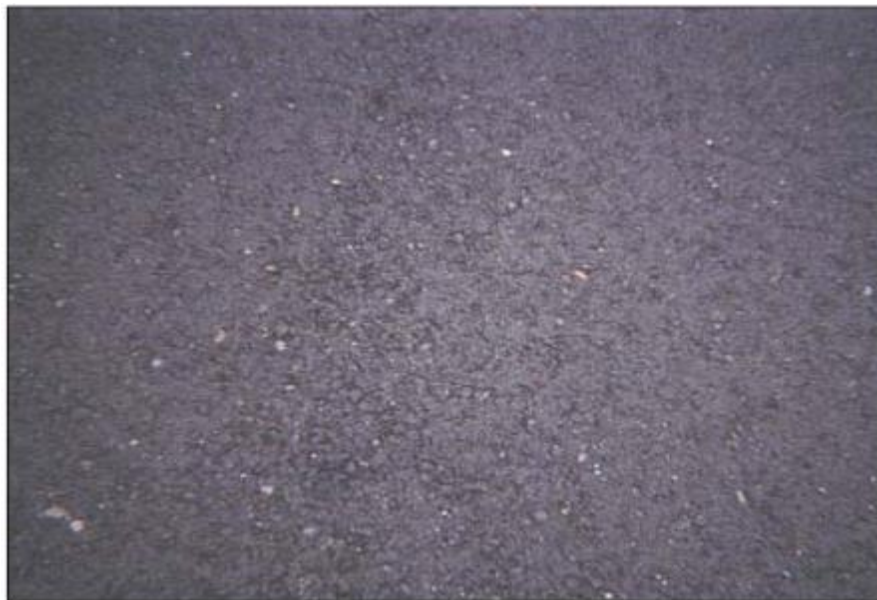
Figure 5. Photo. Dense graded HMA with closed surface texture.
