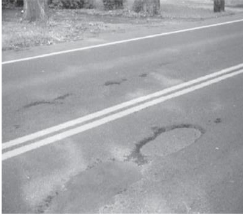
Figure 40. Photo. Delamination of Surface Layer
