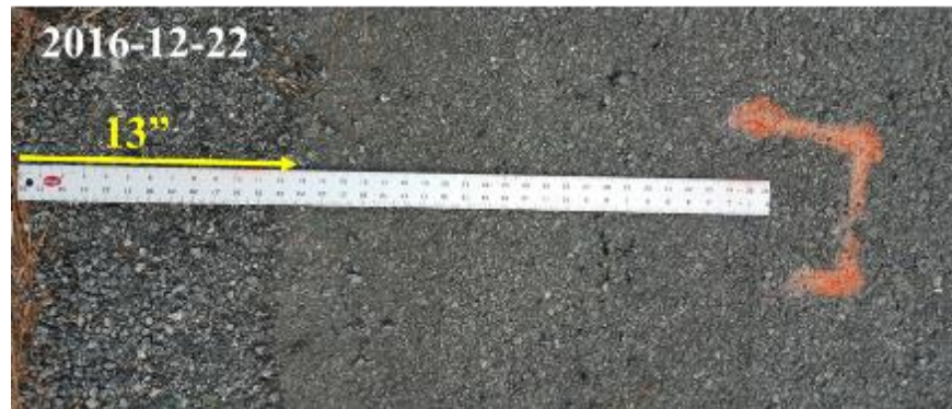
Figure 197. Photo. Width of Aggregate Loss Area along the Shoulder of Site 1
