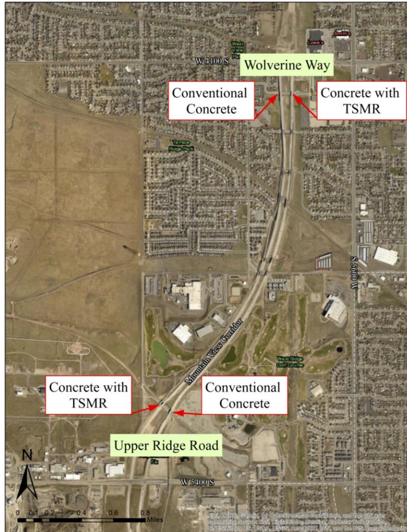
Figure 3-1 Bridge locations and concrete types.
