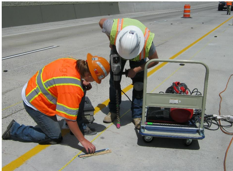
Figure 3-13 Concrete sampling for chloride concentration testing.
