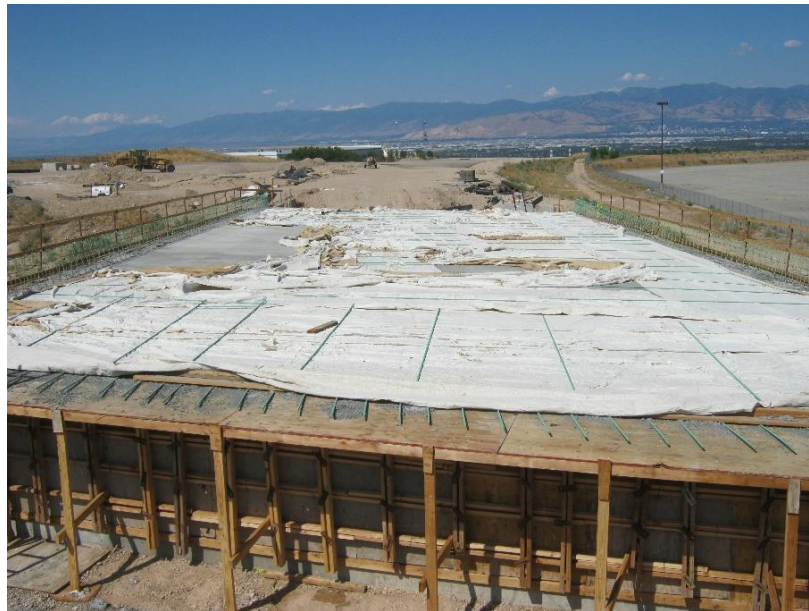
Figure 3-4 Covered bridge deck during curing.
