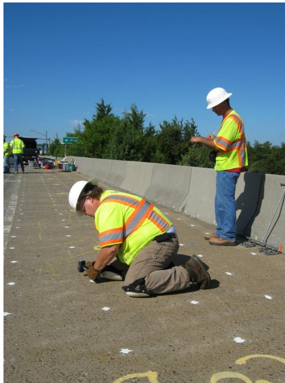
Figure 2-13 Bridge deck sounding with a hammer.
