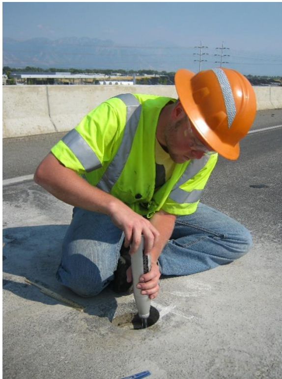
Figure 3-20 Schmidt rebound hammer testing.
