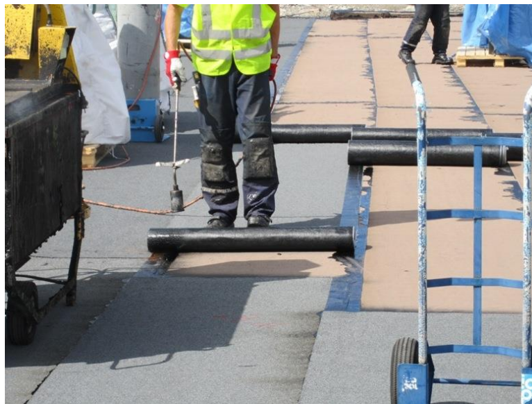
Figure 2-39 Preformed membrane application process.
