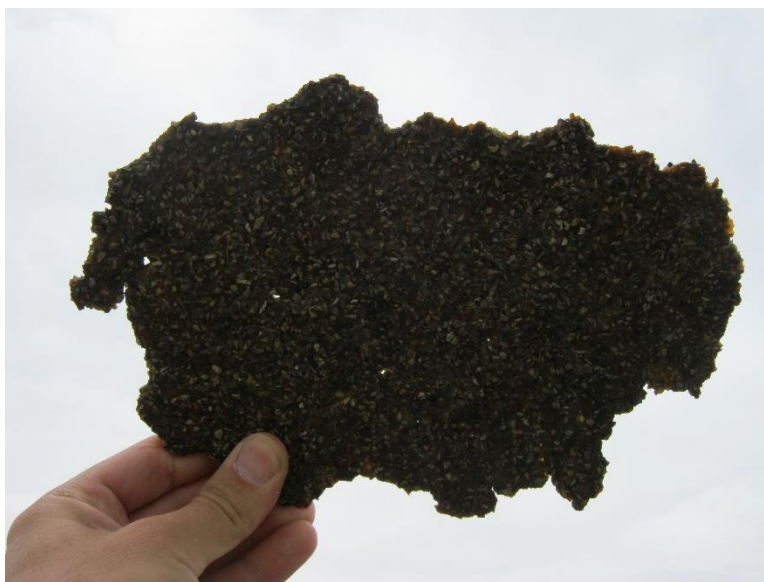
Figure 4-8 Polymer overlay deterioration.
