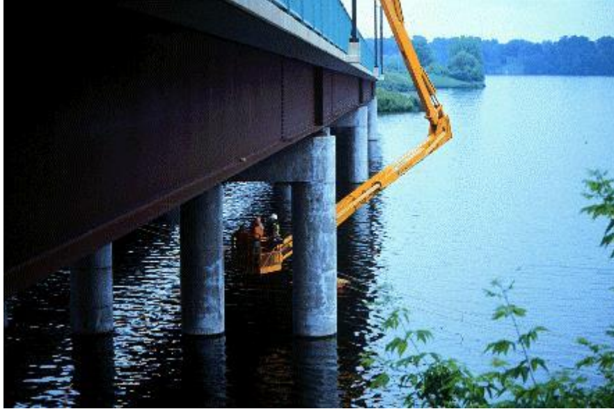
Figure 2-35 Visual inspection of a reinforced concrete bridge deck (Hema et al. 2004).
