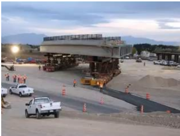
Figure 2-49 Movement of a bridge using mobile transporters.
