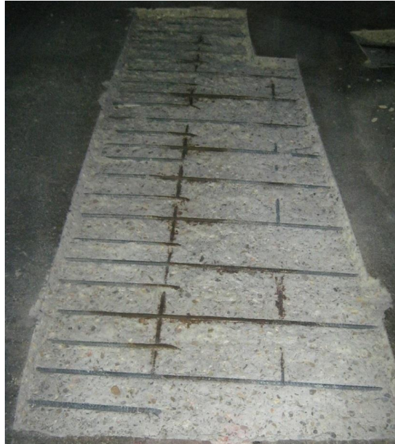
Figure 2-43 Cover concrete removal.
