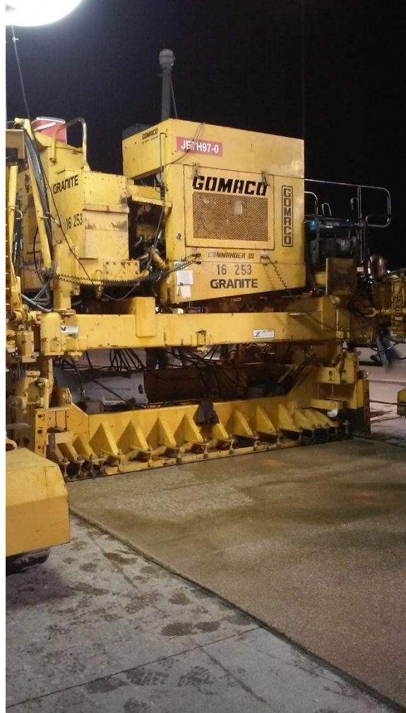
Figure 2-38 PPC overlay placement.
