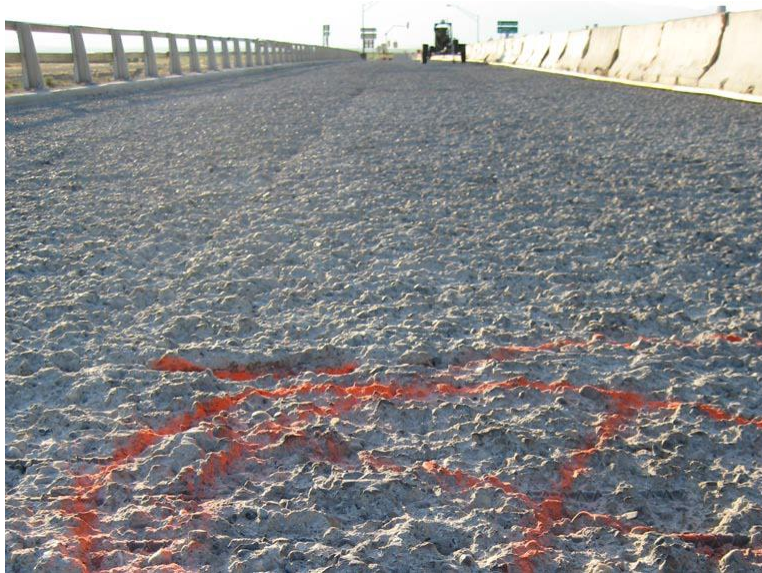
Figure 2-41 Surface prepared for concrete overlay (Nolan 2008).
