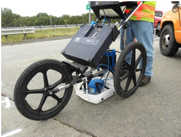
Figure 2-10 GPR testing of a bridge deck.
