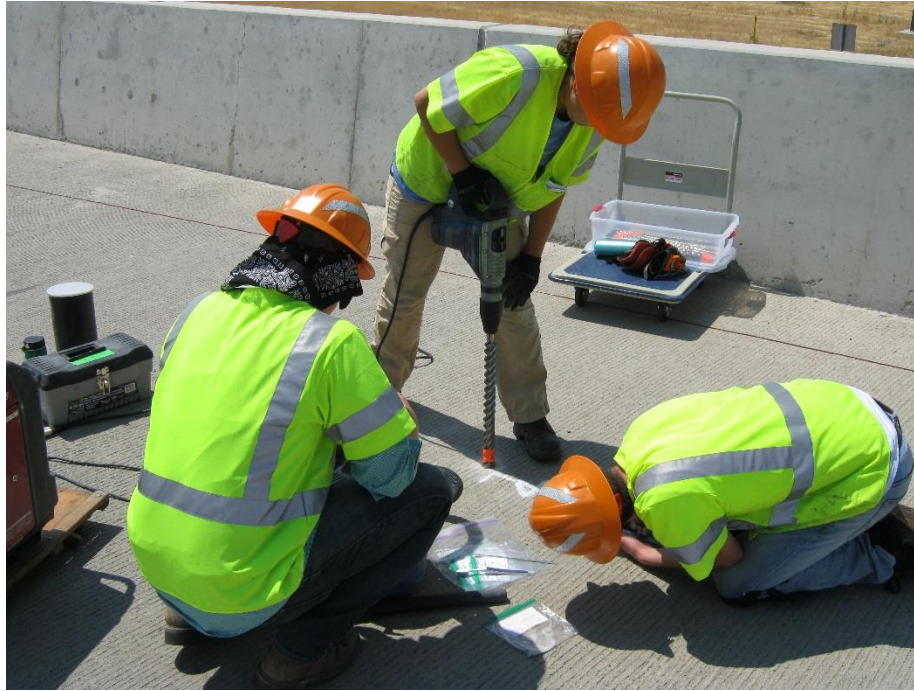
Figure 2-2 Concrete powder sampling for chloride concentration testing.
