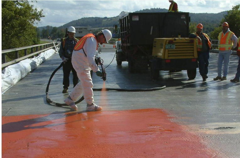
Figure 2-40 Spray-applied membrane application process (Bridge Preservation 2016).
