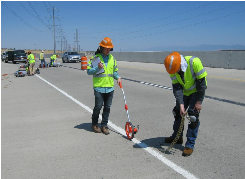
Figure 2-1 Chain dragging of a concrete bridge deck.
