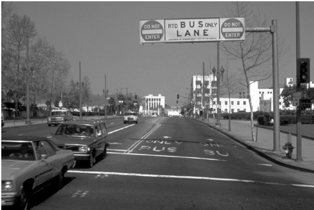
Figure 7. Contraflow Bus-only Lane on Spring Street in Downtown Los Angeles.
