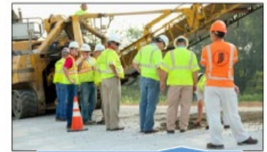
IMI and E&B Paving
