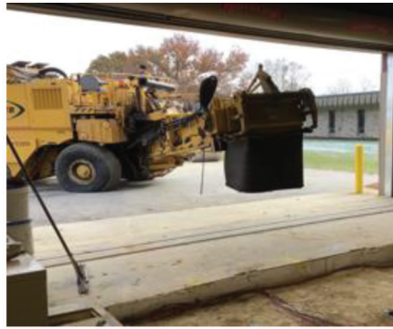
(a) Asphalt base construction (material transfer)
