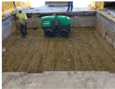
(b) Subgrade soil compaction
