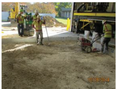
(e) Mixing operations during subgrade stabilization
