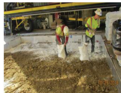
(d) Lime addition during subgrade stabilization
