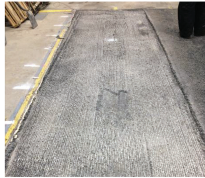
(b) Lane 4 surface milled-off
