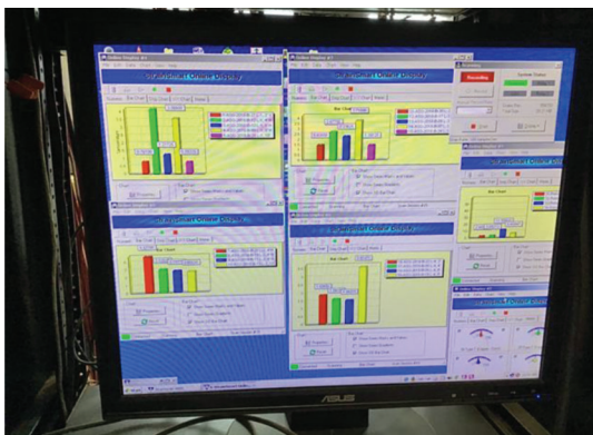
Figure 3.13 Monitoring of pavement sensors during repaving operations.
