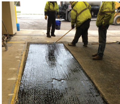
(c) Tack coat application
