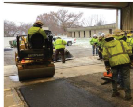
(f) Compacting operations
