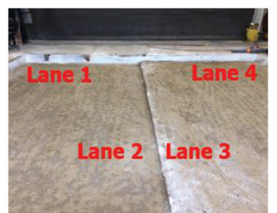
(f) Subgrade finished surface
