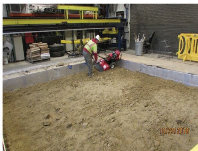
(c) Scarification and compaction of stabilized soil
