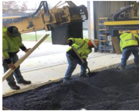
(b) Manual spreading of asphalt base material
