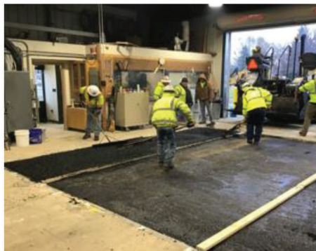
(e) Surface course paving operations (Lane 1)
