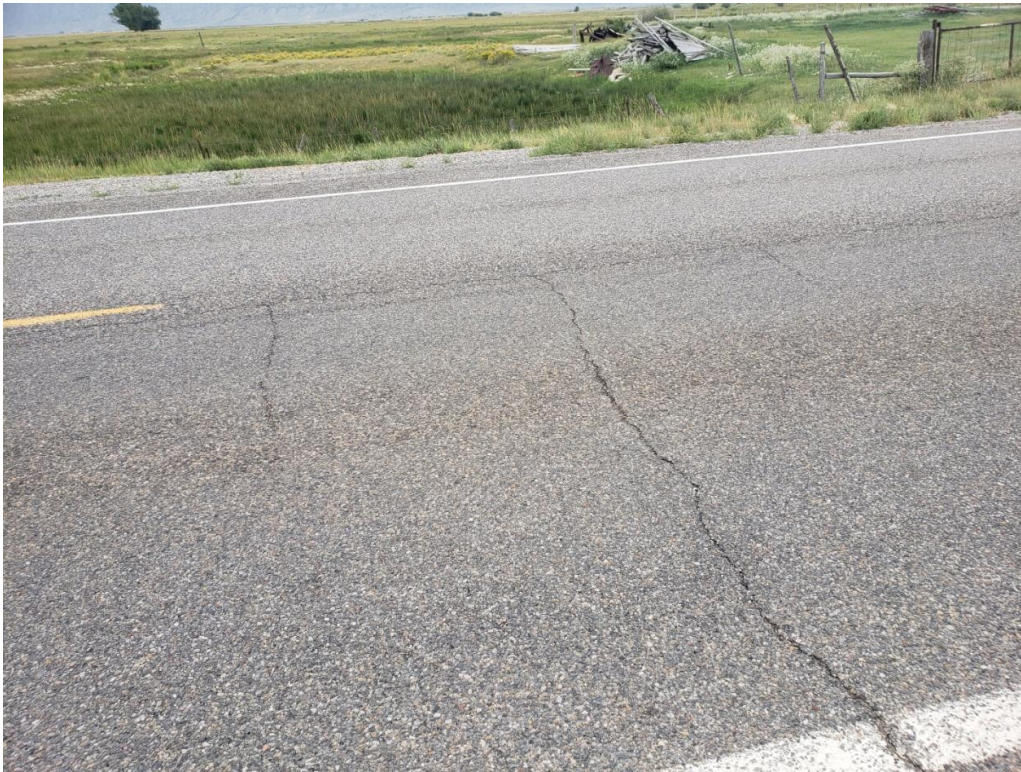
Figure 5-2 Section UT-03 Showing Thermal and Reflective Cracking
