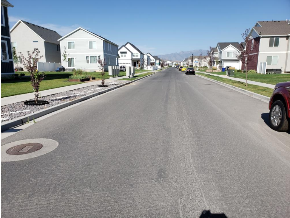
Figure 5-5 Section UT-07 Showing No Distresses
