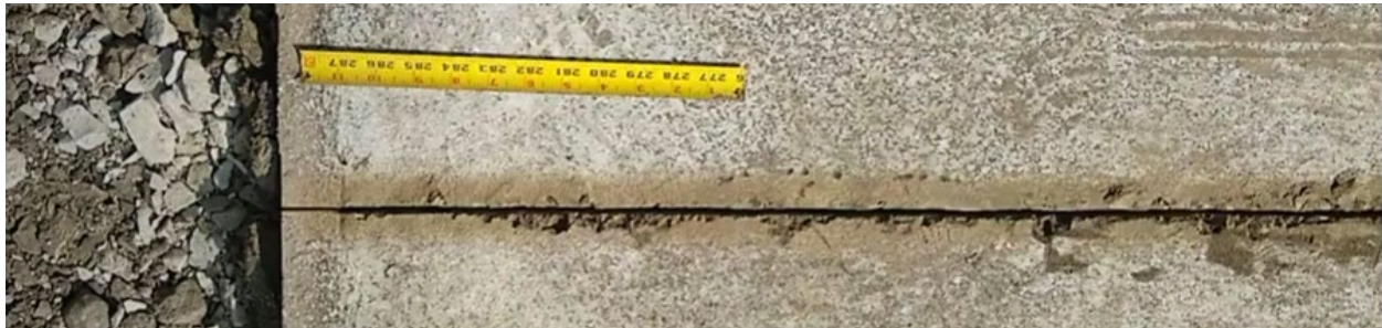
A. Control mix: Saw cut after 4 hours 25 minutes
