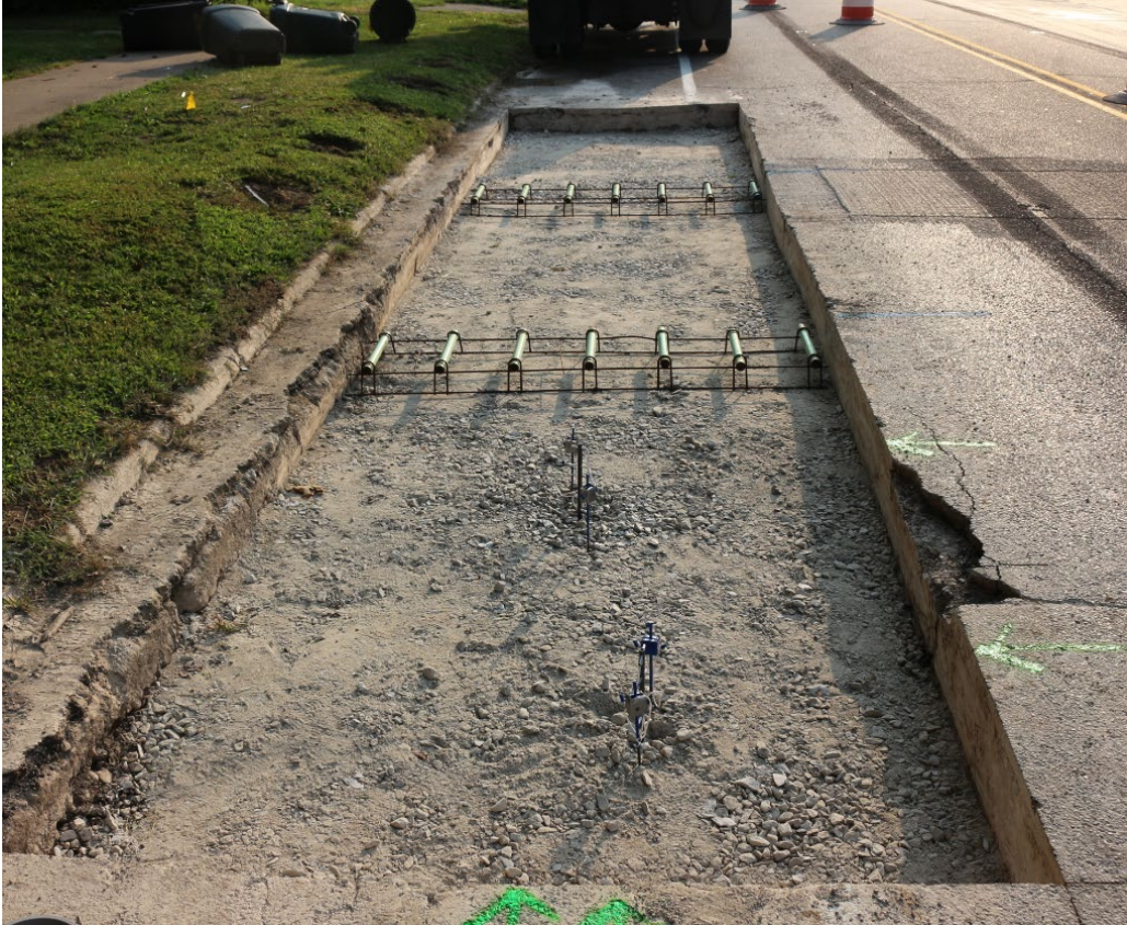
A. Thermal sensors installed in the field test section
