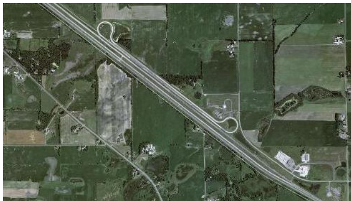
Figure 21. Aerial View of MnROAD Test Facility
