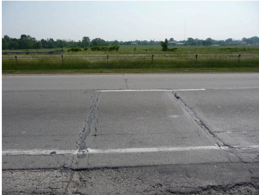
Figure A.3 Example Inverted-T patching.
