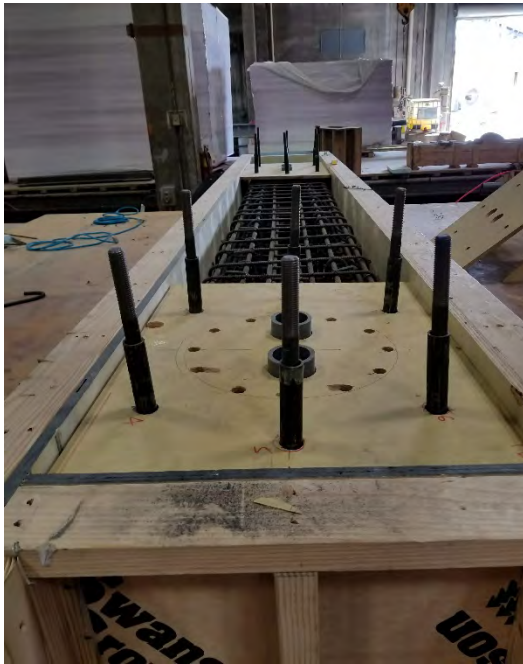
Figure 3.7 Construction details of the cap-beam
