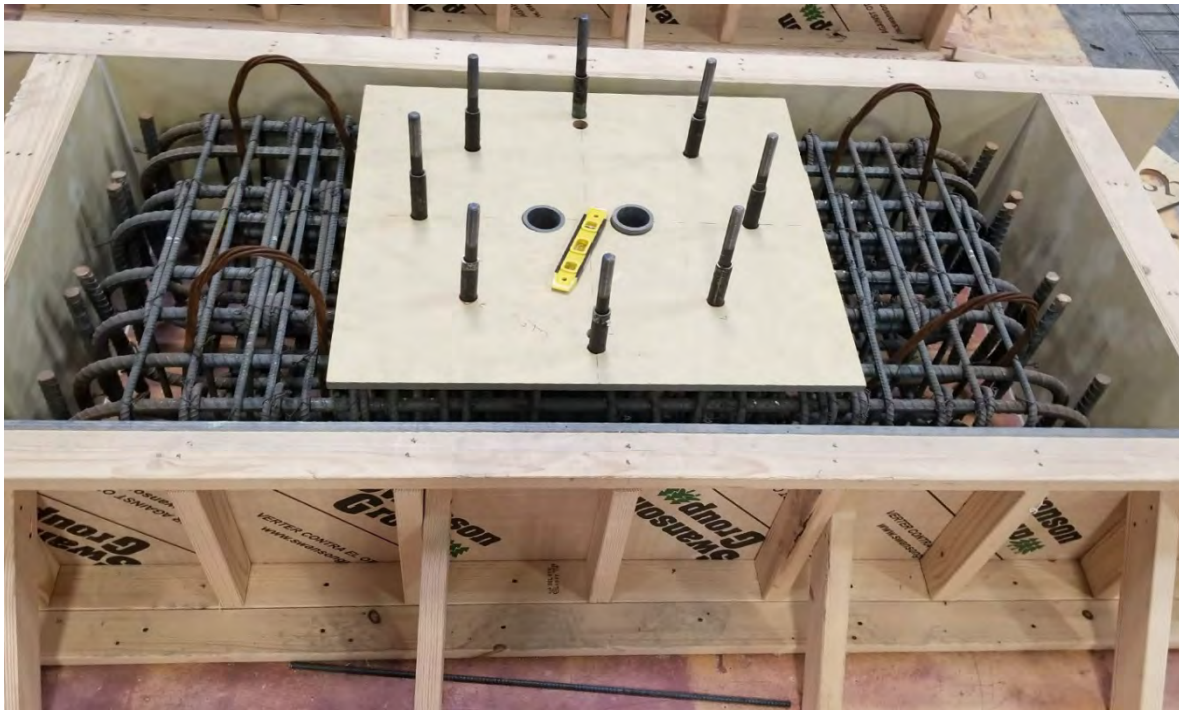
Figure 3.15 Construction details of the footing
