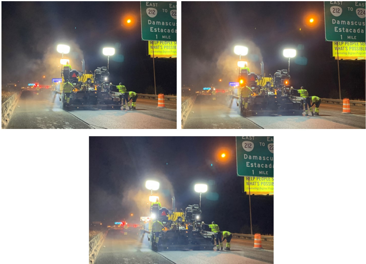
Figure 3.3: Only balloon lights on (top-left), amber lights on (top-right), and white lights on (bottom) (case study 2)
