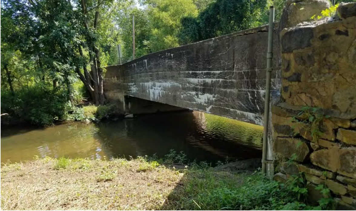
Figure C-3: Inlet of structure. PennDOT photo.
