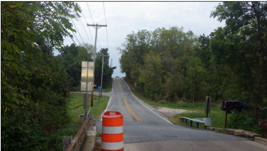
Figure A-2: Baker Road Left Approach. Credit: PennDOT
