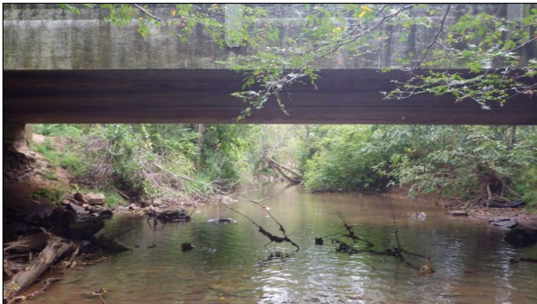
Figure A-3: Baker Road Bridge – Looking Downstream. Credit: PennDOT
