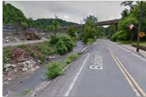
Streets Run Road in Allegheny County Credit: PennDOT
