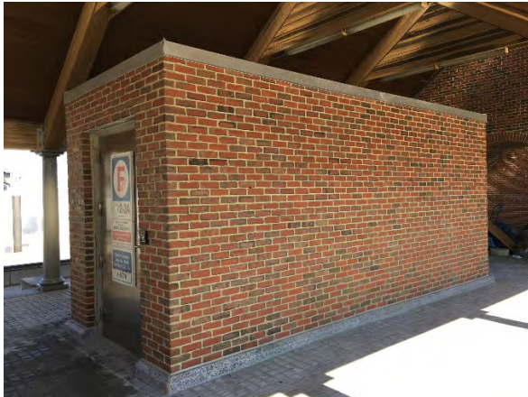
Figure 17 – Long Wharf Headhouse Complete (Credit: MassDOT)
