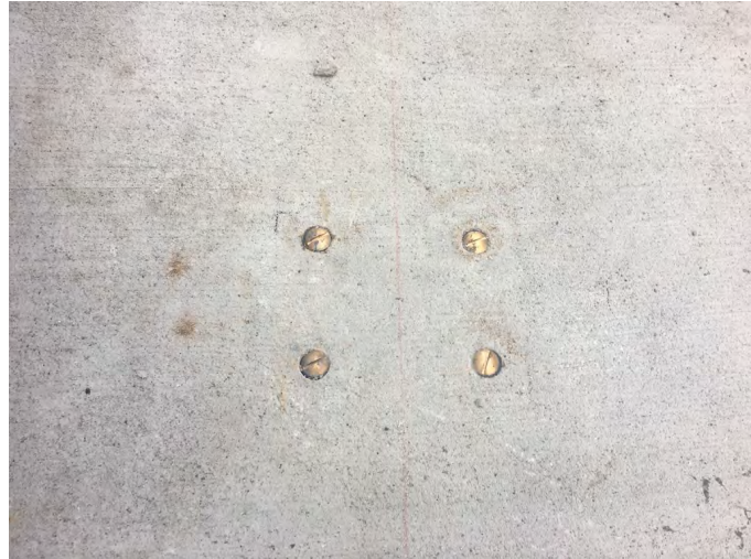
Figure 14 - Blanking Bolts at Post Location when Posts not Deployed (Credit: MassDOT)
