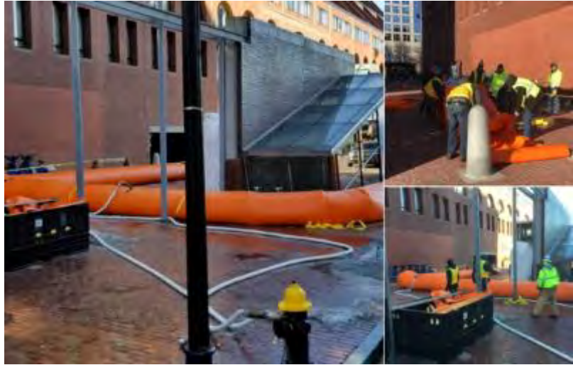
Figure 12 - Water-Filled Flood Barriers During Test Deployment by MBTA in February 2019 (Credit: MassDOT)
