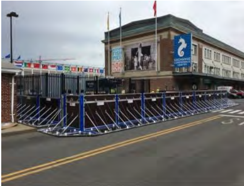
Figure 11 - Example of Deployed Composite Flood Panels (Credit: MassDOT)
