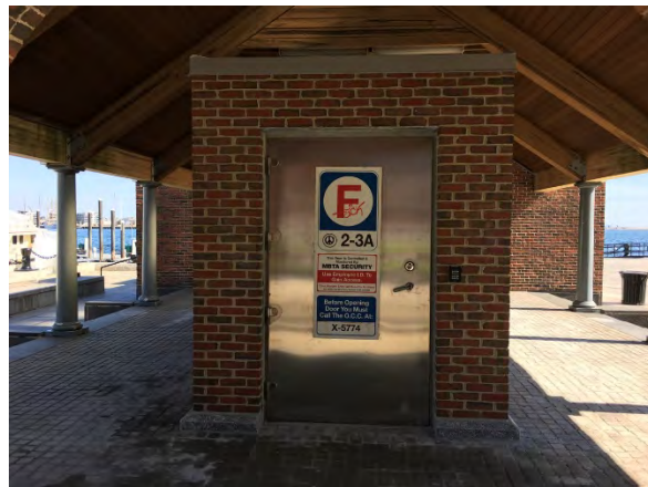
Figure 18 – Long Wharf Flood Door – Exterior (Credit: MassDOT)
