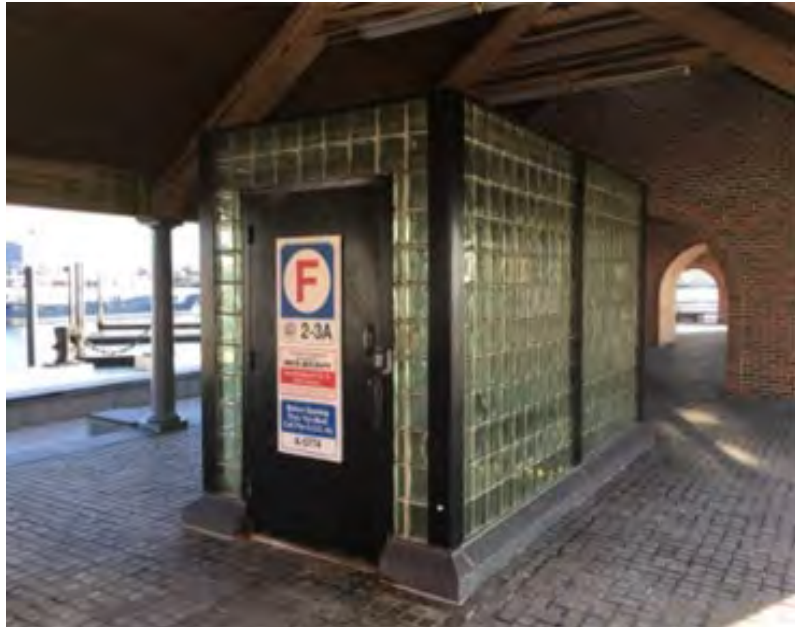
Figure 7 - Long Wharf Blue Line Tunnel Emergency Egress Kiosk (Credit: MassDOT)
