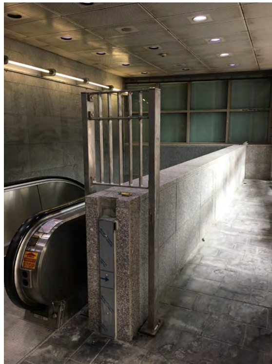
Figure 24 – Marketplace Center Concrete Floodwall (Credit: MassDOT)
