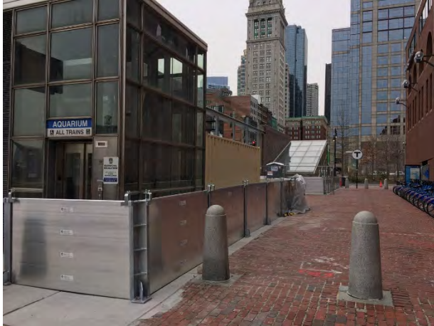
Figure 21 – East Headhouse Flood Barriers (Credit: MassDOT)
