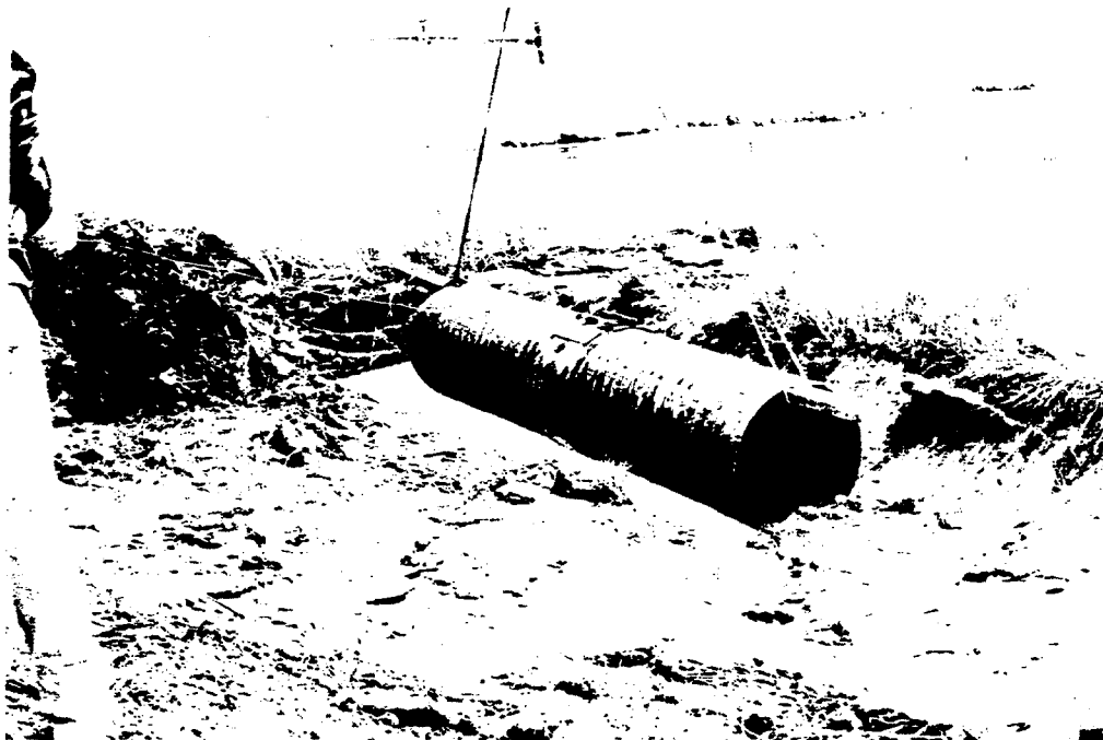
Figure B.31.1. The unprotected corrugated steel pipe is lowered into the ditch. (8)
