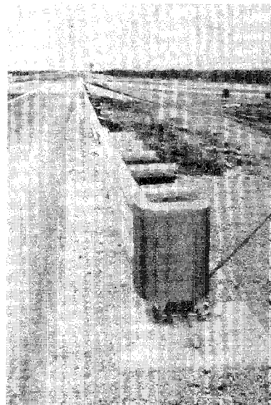
Slide No. 6-2-44J Example Slide TREND dual purpose end treatment
