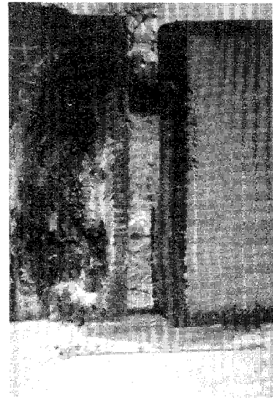
Slide No. 3-2-27 Example Slide Marine borer damage to a timber pile
