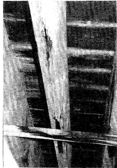
Slide No. 5-2-61 Example Slide Beam No. 7 at West Abutment
