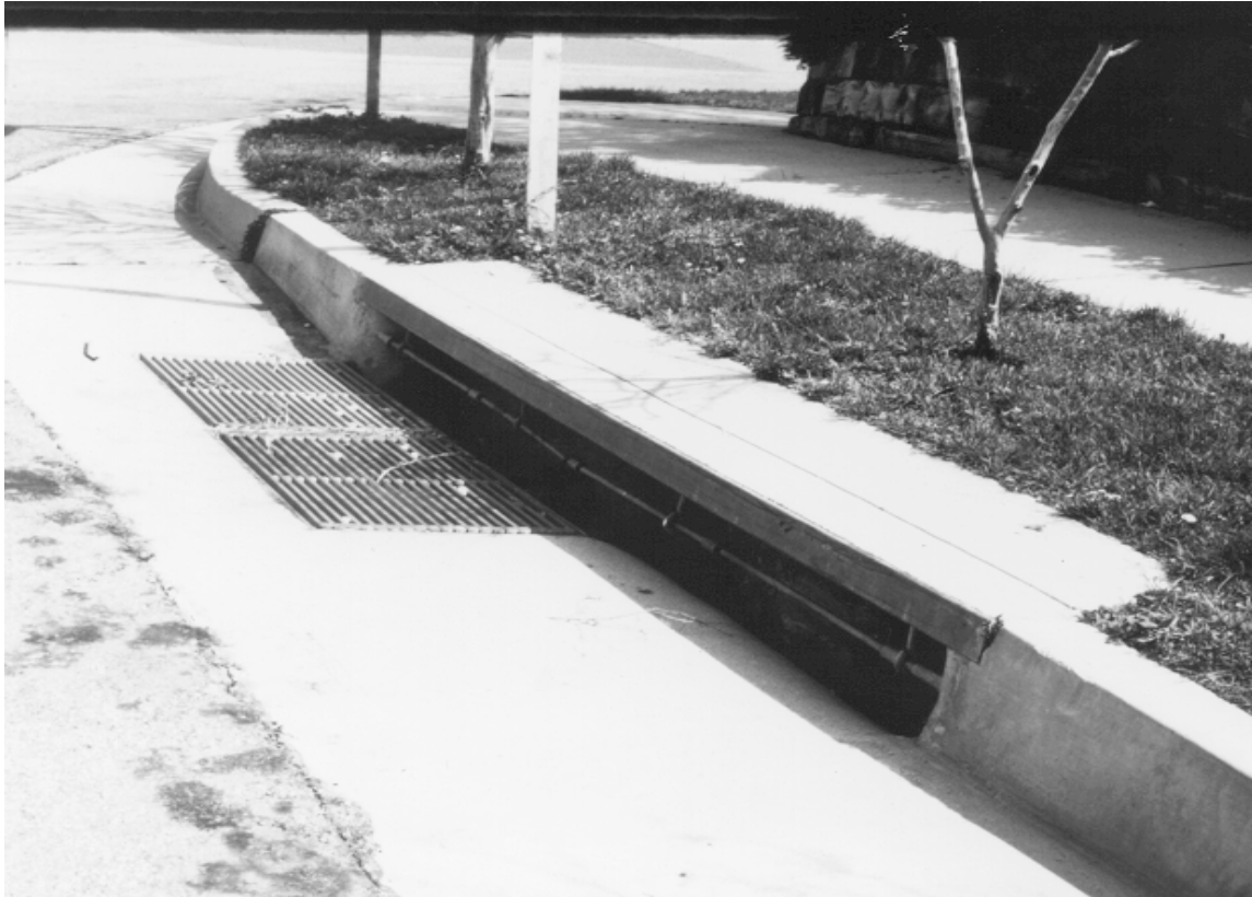
Figure 4-16. Sweeper combination inlet.
