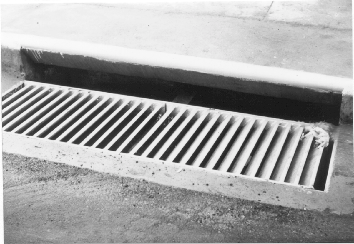
Figure 4-15. Combination curb-opening, 45 degree tilt-bar grate Inlet.
