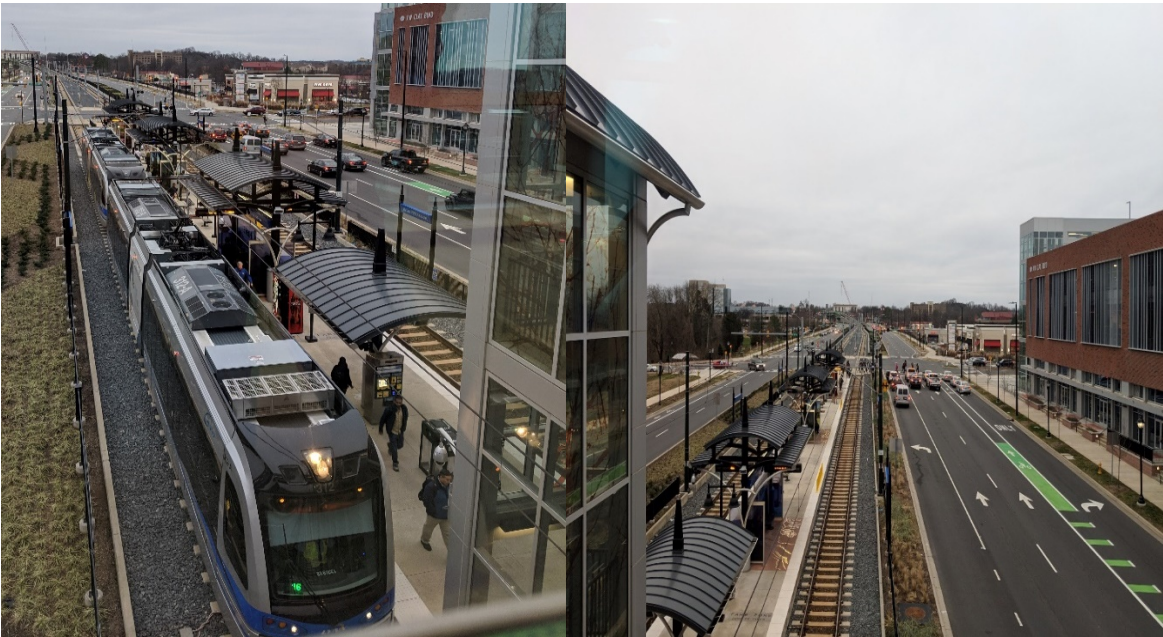
Figure 14. Interaction of the LRT System with the Moving Traffic, On-street Bicycle Lane, and Pedestrian Crosswalks
