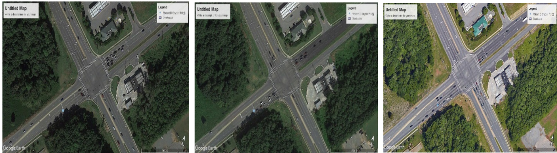
Figure 11. N Tryon St & E Mallard Creek Church Rd Intersection: 2016, 2017, & 2018 (Left to Right)
